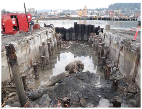
Photograph 39: Central Waterfront barge ramp demolition at the Maple Street Bulkhead. Facing south.
