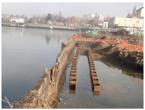
Photograph 4: South shoreline during removal of the steel sheetpile bulkhead. Facing east.
