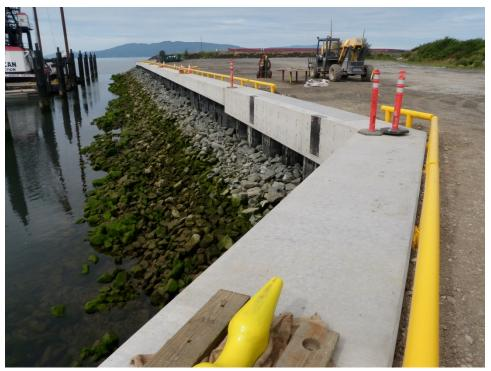
Photograph 48: Central Waterfront: WCWW concrete pilecap. Facing west.
