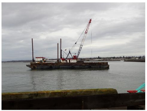
Photograph 36: BST capping operations. Facing northeast.
