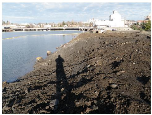
Photograph 5: South shoreline following removal of the steel sheetpile bulkhead and timber bulkhead. Facing east.
