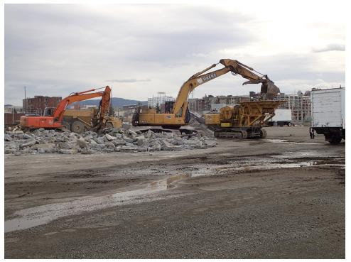
Photograph 17: Former GP West SSA concrete reduction and sorting. Facing south.
