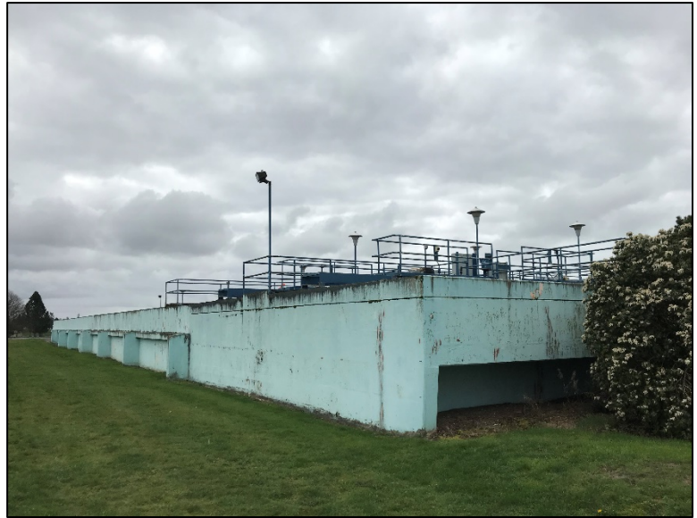
Decommissioned Sedimentation Basin facing south, March 2018
