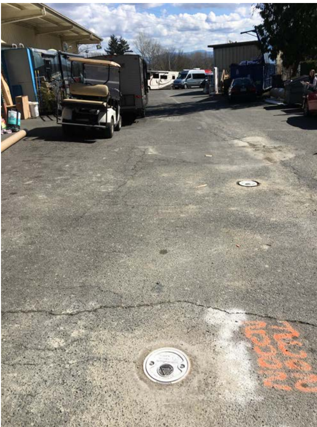
Photo 4: WSDOT recently installed five groundwater monitoring wells on the property.
