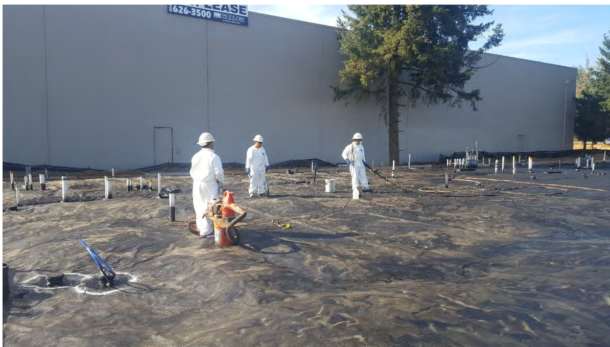
APPLICATION OF LOW-PERMEABLE MEMBRANE AND SMOKE TEST SETUP. PHOTOGRAPH TAKEN FACING SOUTHWEST.
