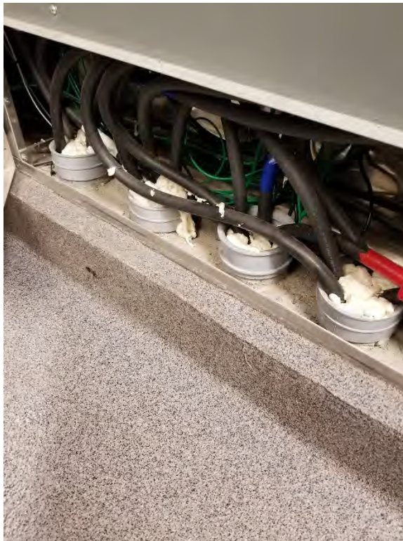
CONDUIT SEALS IN INTERIOR ELECTRICAL PANEL.
