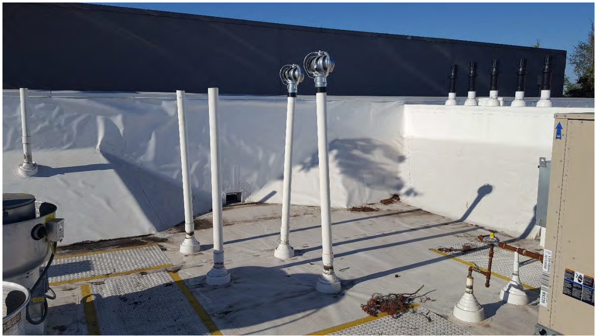
VENT RISERS WITH WIND TURBINES ON WEST SIDE OF BUILDING. PHOTOGRAPH TAKEN FACING SOUTH.
