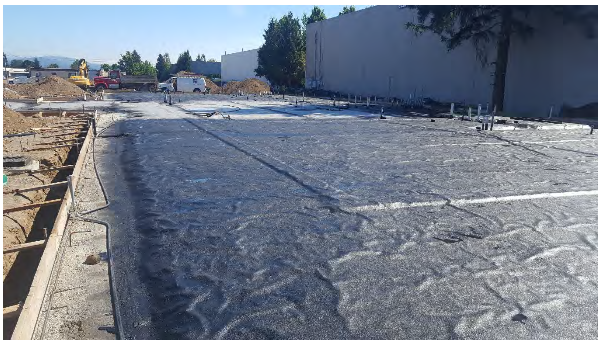
APPLICATION OF LOW-PERMEABLE MEMBRANE. PHOTOGRAPH TAKEN FACING EAST.
