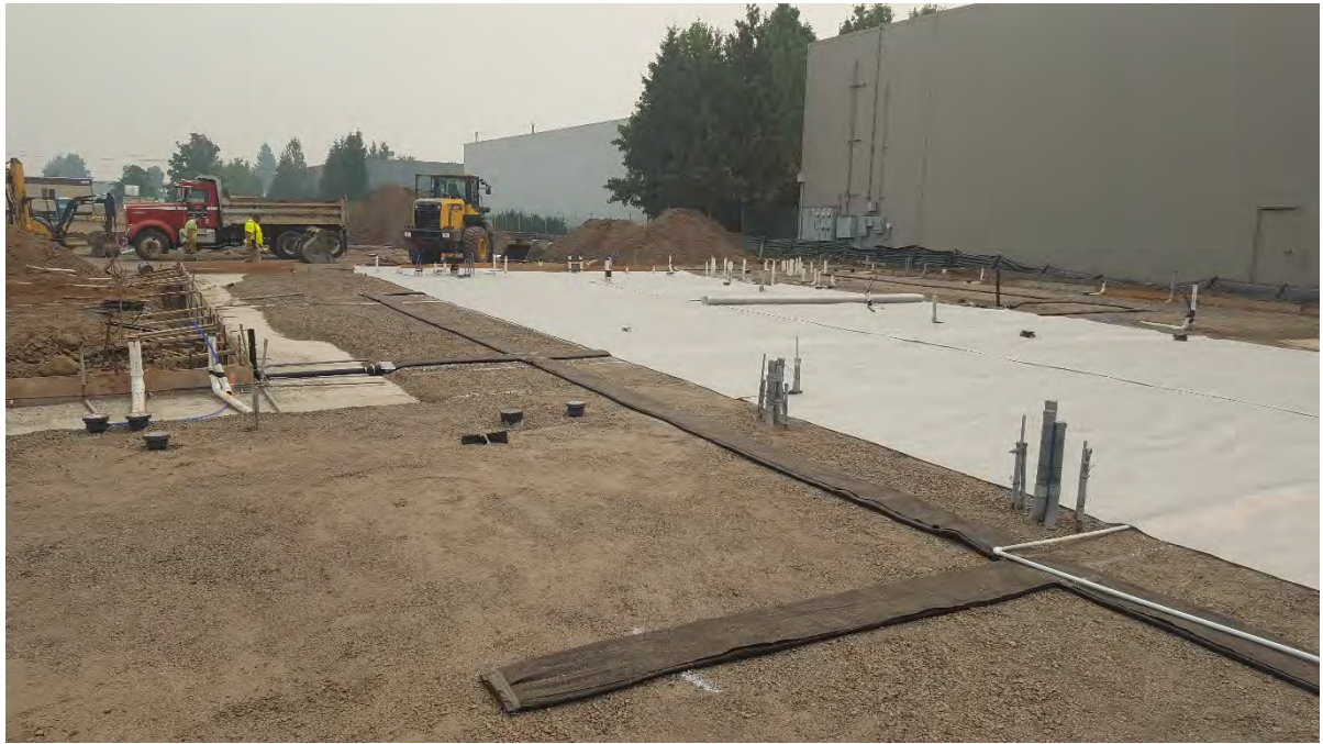
SUB-SLAB VENT PIPE LAYOUT. PHOTOGRAPH TAKEN FACING SOUTHEAST.
