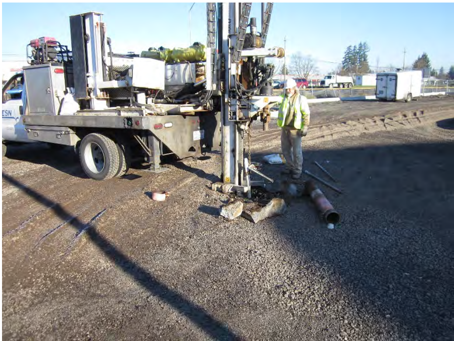
ABANDONMENT OF MONITORING WELL MW-2. PHOTOGRAPH TAKEN FACING NORTH.
