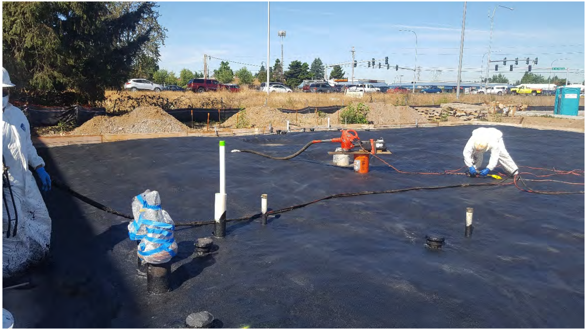
LOW-PERMEABLE MEMBRANE AND SMOKE TEST SETUP. PHOTOGRAPH TAKEN FACING NORTHEAST.
