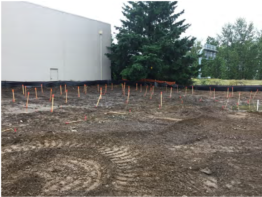
STAKING FOR ENGINEERED AGGREGATE PIERS. PHOTOGRAPH TAKEN FACING SOUTHWEST.
