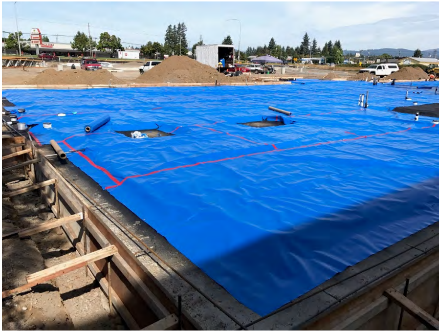
PROTECTIVE SHEETING OVER LOW-PERMEABLE MEMBRANE. PHOTOGRAPH TAKEN FACING NORTH.
