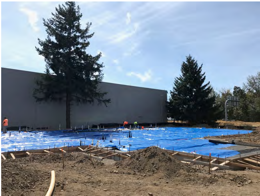
PROTECTIVE SHEETING OVER LOW-PERMEABLE MEMBRANE. PHOTOGRAPH TAKEN FACING SOUTHWEST.
