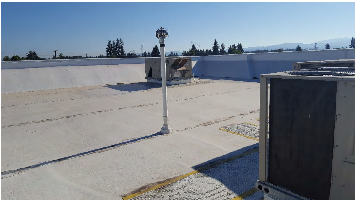
VENT RISER WITH WIND TURBINE ON EAST SIDE OF BUILDING. PHOTOGRAPH TAKEN FACING SOUTHEAST.
