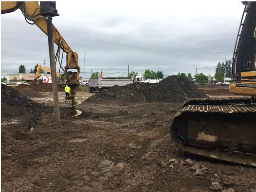
AUGER FOR ENGINEERED AGGREGATE PIERS. PHOTOGRAPH TAKEN FACING NORTH.
