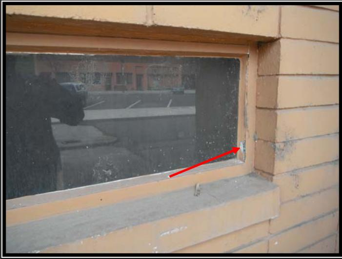
**Image 7:** Gray window putty was identified through laboratory analysis to be an **ACM**
