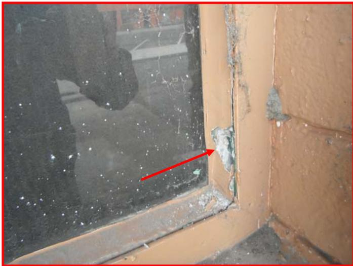
**Image 8:** Gray window putty was identified through laboratory analysis to be an **ACM**
