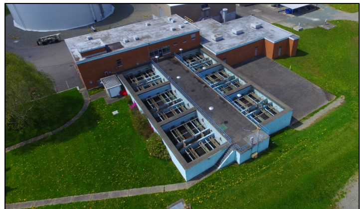
Decommissioned Filtration Basin
