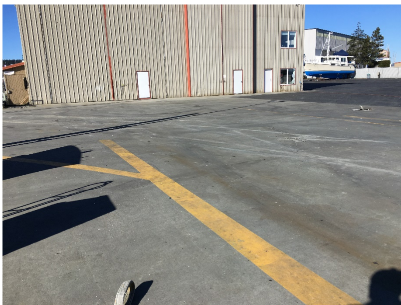
Figure 2 Description: Yellow lines depict limits of pressure wash pad. Grade from yellow lines slopes in toward the center.
