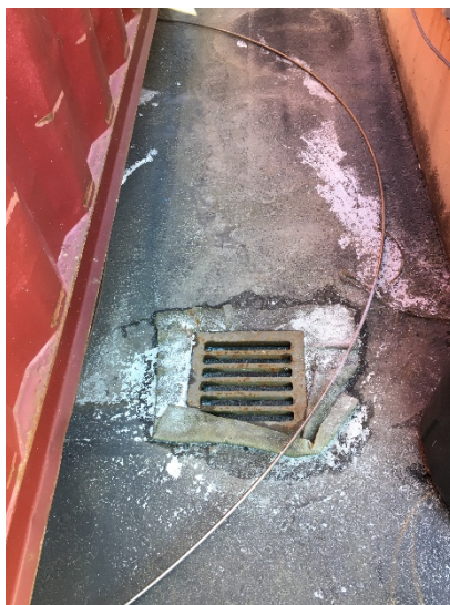
Figure 19 Description: White paint staining on geotextile fabric, but not on catch basin grate, in the southwest corner of the facility. This catch basin is located within 10-feet of the paint mixer.
