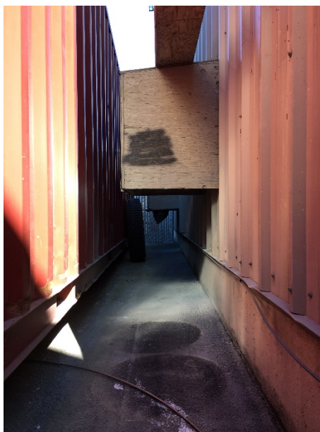
Figure 26 Description: Particulate fall out from inside exhausts depositing on the pavement between the building and paint storage-shipping container. The absence of dust suggests two barrels were previously stored here and have since moved.
