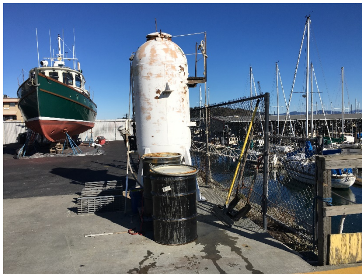
Figure 5 Description: Modified 500-gallon propane tank to treat pressure wash water prior to discharge to City of Anacortes POTW. The tank is within 5-feet of the marine shoreline. No curbing present on boundary between tank and marine waters.
