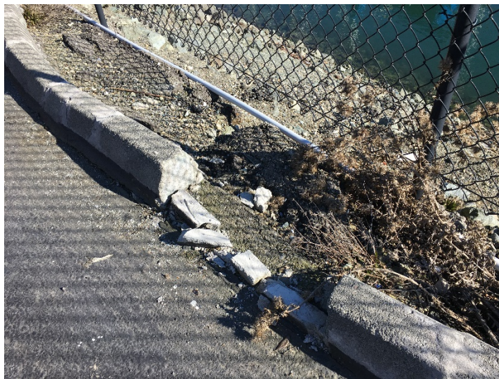
Figure 9 Description: Broken, missing curbing and associated rill on slope to marine waters.
