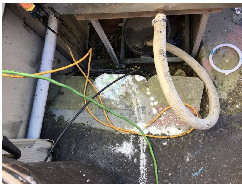
Figure 18 Description: White paint residue from past spill on top and side of trench wall.
