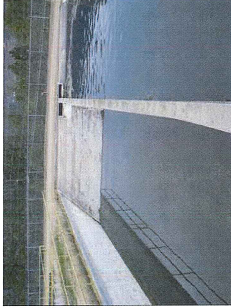
Photo 13: Settling basin in effluent treatment system. During normal operation the generating station only uses one of two basins.
