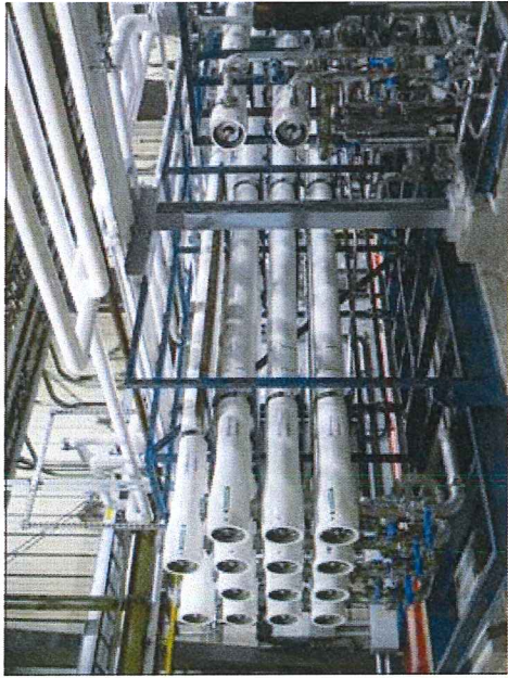
Photo 5: Reverse osmosis units used to treat incoming supply water.
