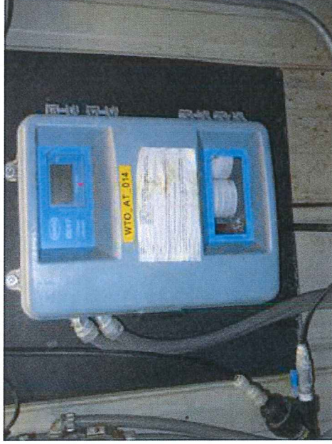
Photo 9: Automatic effluent residual chlorine analyzer.
