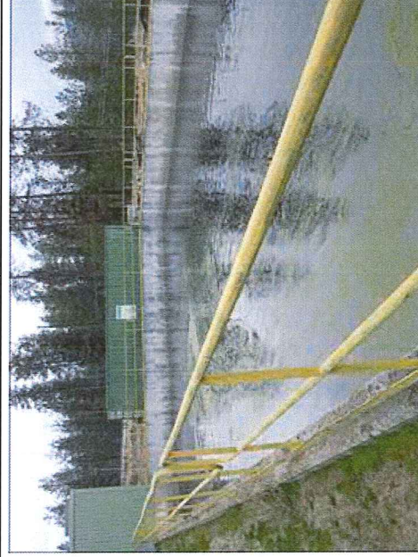
Photo 15: Effluent retention basin. From this basin, pumps transfer the water into the effluent discharge line.
