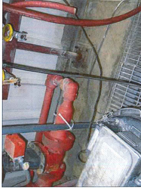
Photo 11: Effluent composite sampler and intake line.
