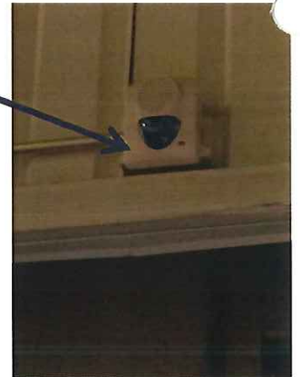
Ammonia Alarm above the Cooler doorway
