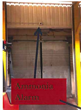
Ammonia Alarm above the Cooler doorway
