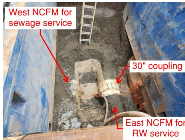
Figure 3: Exposed East and West NCFMs
