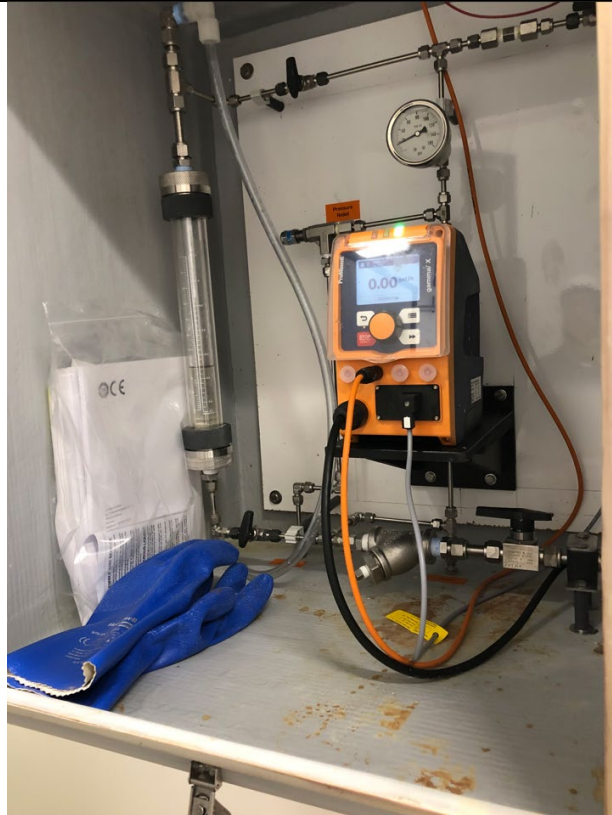
Photo 1: View inside COW water treatment tank. Biofilm is the white material forming on the surfaces of the tank.
