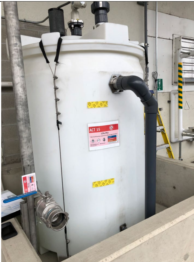
Photo 4: PAA storage tank located outdoors. The carbon filter is located on the top of the tank.
