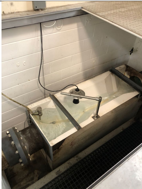
Photo 6: COW water effluent flow meter and discharge point from facility.
