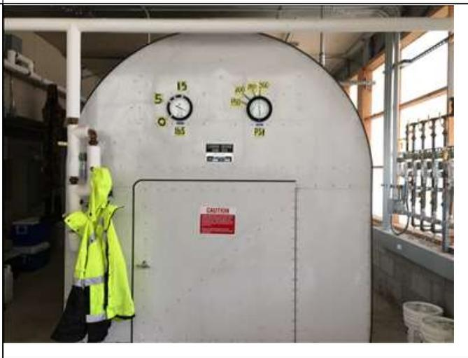
A photograph of a large, white, cylindrical carbon dioxide storage tank. The tank has two pressure gauges on top, one labeled '15' and the other '150'. A red 'CAUTION' label is visible on the front door. A yellow safety vest is hanging on the left side of the tank.     | <p>Carbon dioxide storage tank.</p>                                                                           |
