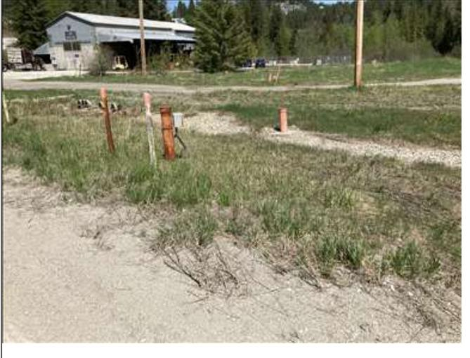
A photograph showing a monitoring well in a field. The well is a vertical pipe with a cap, surrounded by a gravel area. In the background, there is a large white building with a blue roof, possibly a treatment facility, and some trees. | Monitoring well next to the residual treatment pilot.                                       |
