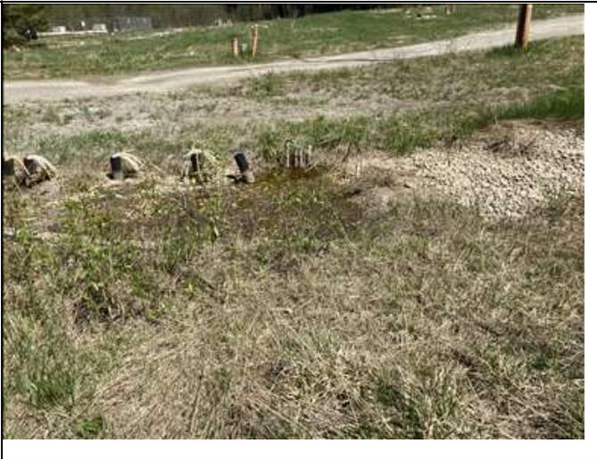
A photograph showing abandoned infrastructure for a carbon dioxide treatment pilot. There are several open pipes protruding from the ground in a field of tall grass. A gravel area is visible in the foreground.                          | Original carbon dioxide treatment pilot abandoned infrastructure. Open pipes in the ground. |
