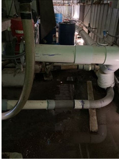
Photo 45. More piping for wastewater flow, leaving DAF.
