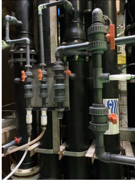
Photo 43. Chemical treatment prior to entering DAF.
