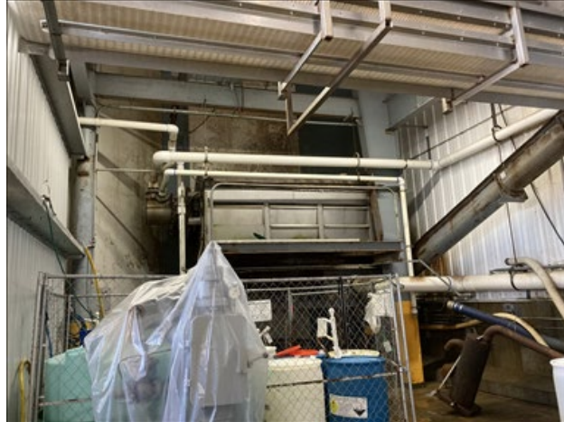
Photo 37. Hydro-sieve in Clear Ocean building.
