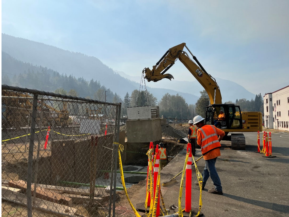
Photograph 19: Replacement of Access Lids.
