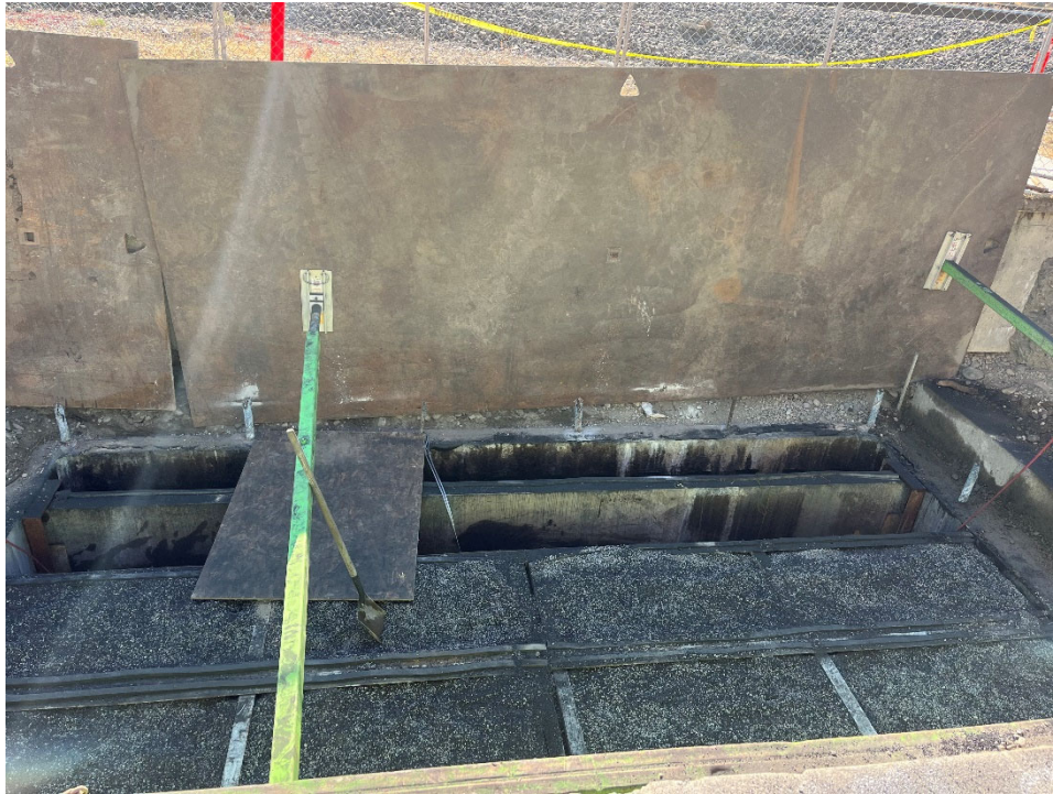
Photograph 15: Replaced GAC/Pea Gravel Material.
