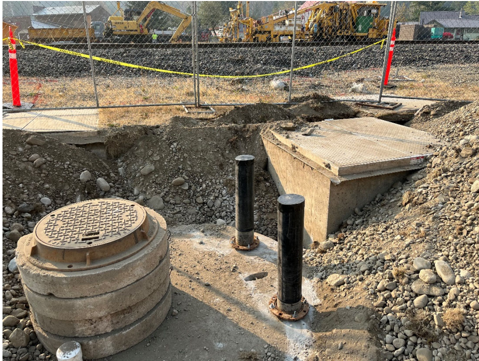
Photograph 25: Exposed Temporary Risers for Wells.
