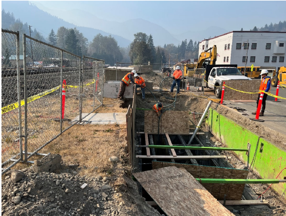
Photograph 11: Vault Dewatering.
