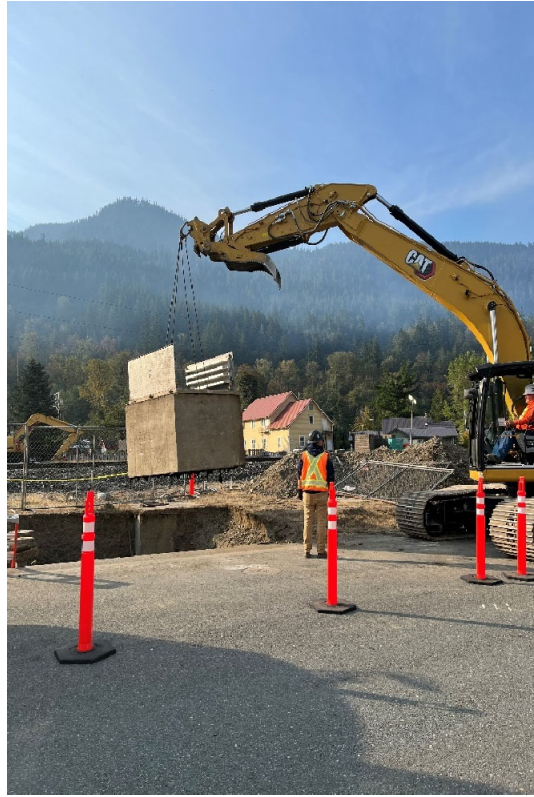
Photograph 3: Removal of Vault Access Hatch.
