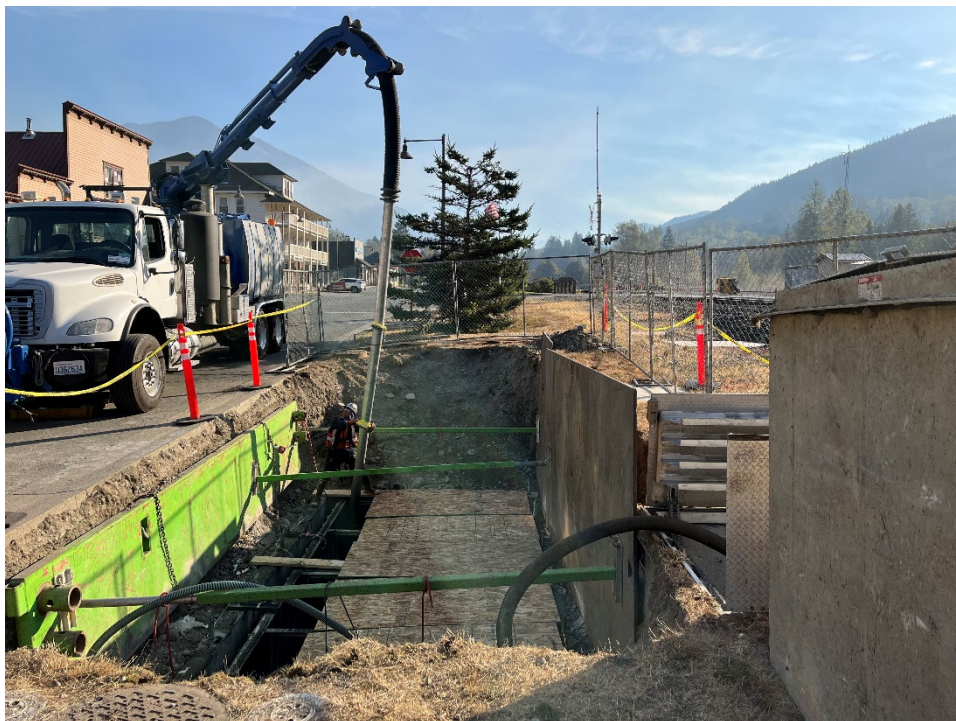
Photograph 12: Removal of Saturated Material with Vector.
