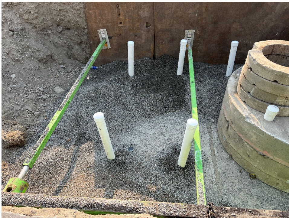
Photograph 22: PVC Covering Anchor Bolts.
