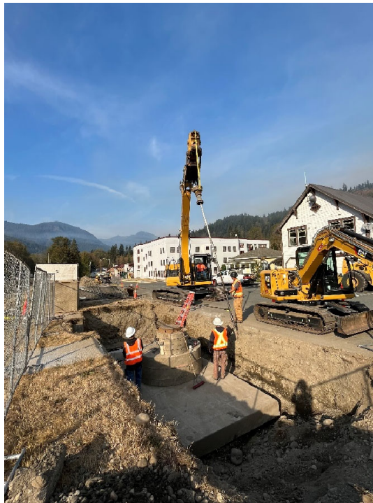
Photograph 4: Removal of Wells.
