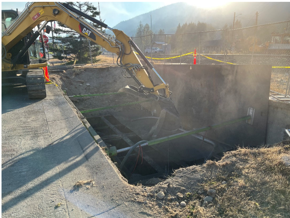
Photograph 14: Placement of GAC/Pea Gravel Material.
