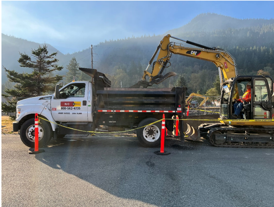
Photograph 13: Mixing of GAC/Pea Gravel Material.
