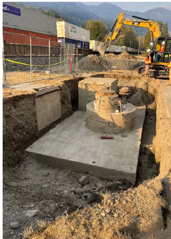
Photograph 2: Excavation to Vault Top.
