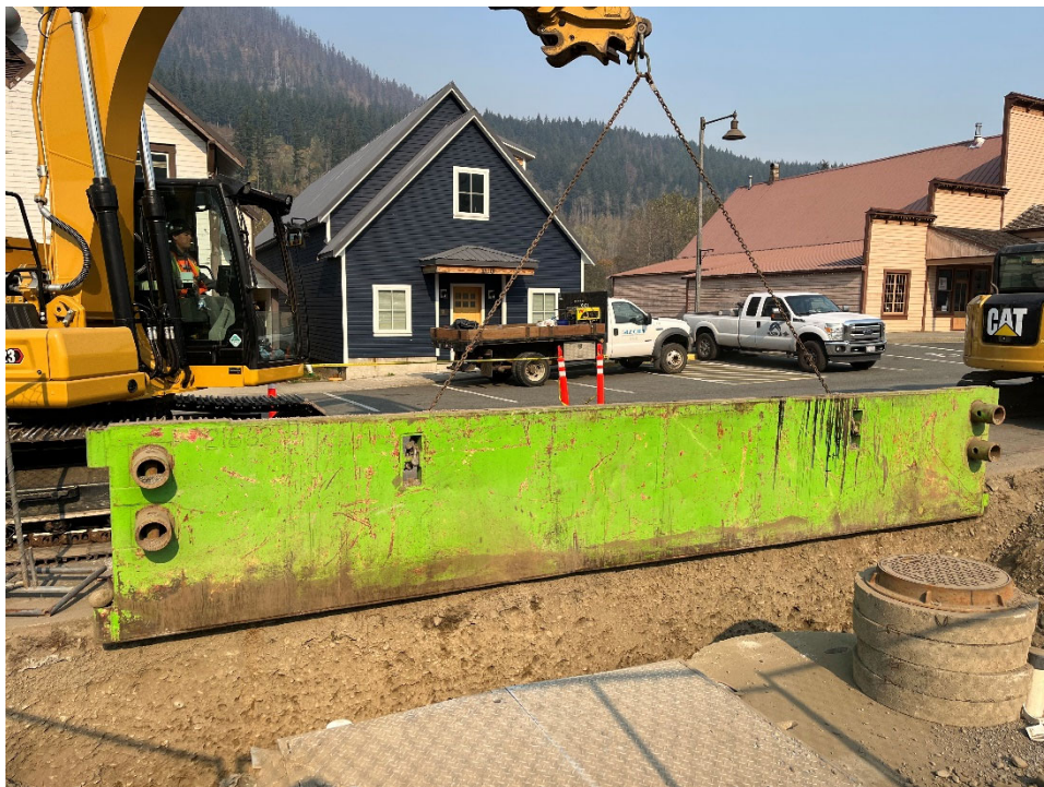
Photograph 24: Removal of Shoring.
