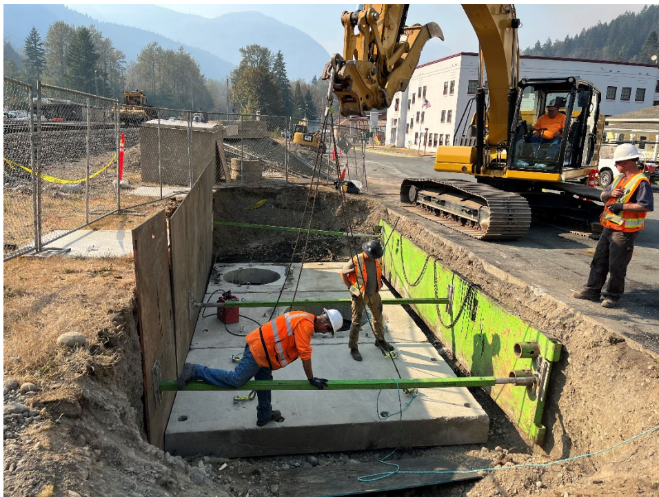
Photograph 18: Reinstalled Vault Lid.
