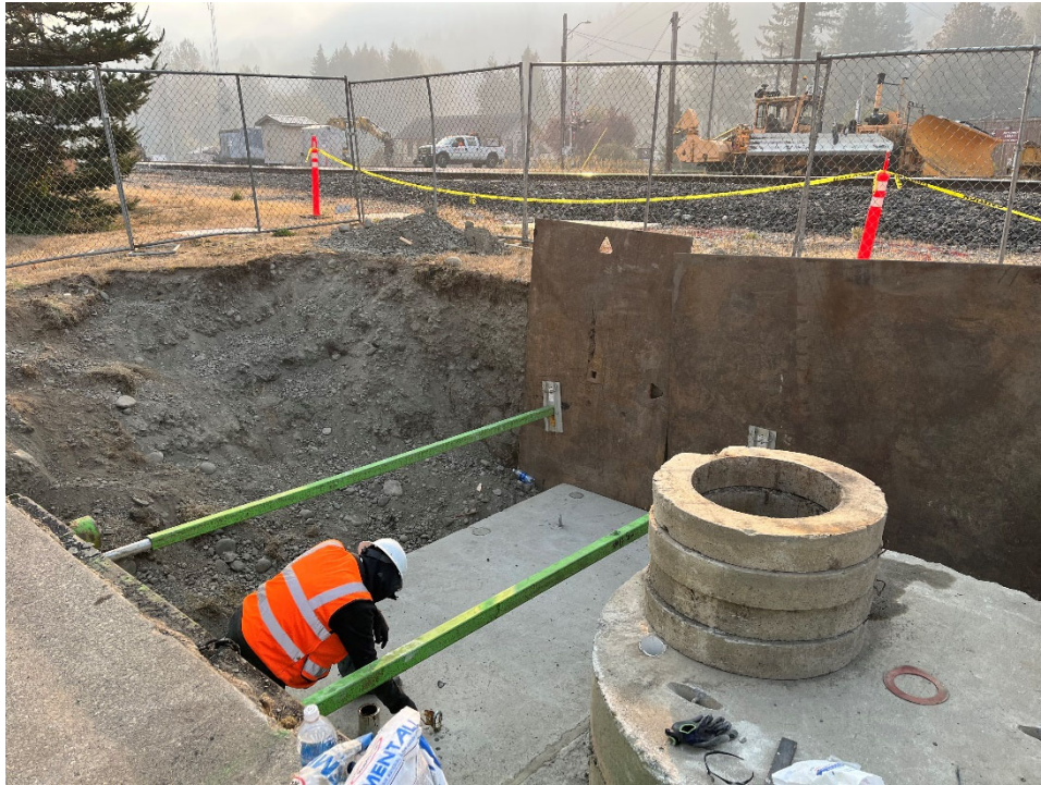
Photograph 21: Grouting Dowel Post Connections.
