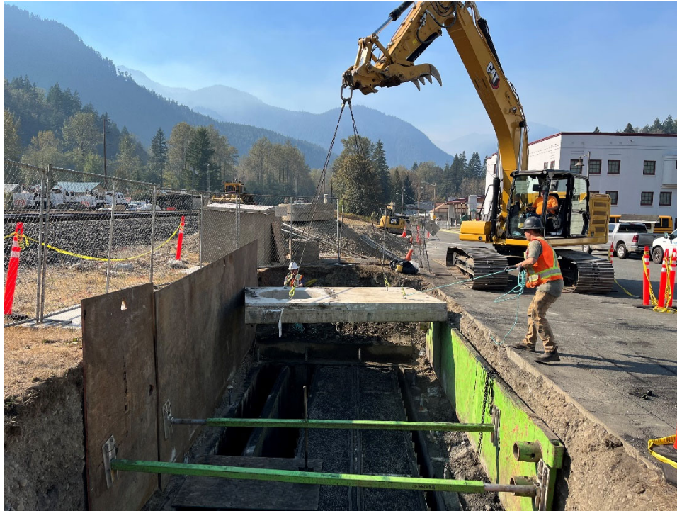
Photograph 17: Reinstallation of Vault Lid.
