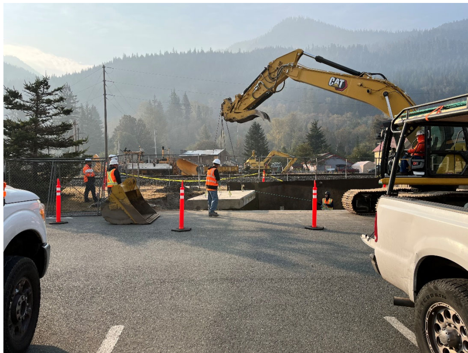
Photograph 6: Lifting of Concrete Vault Lid.
