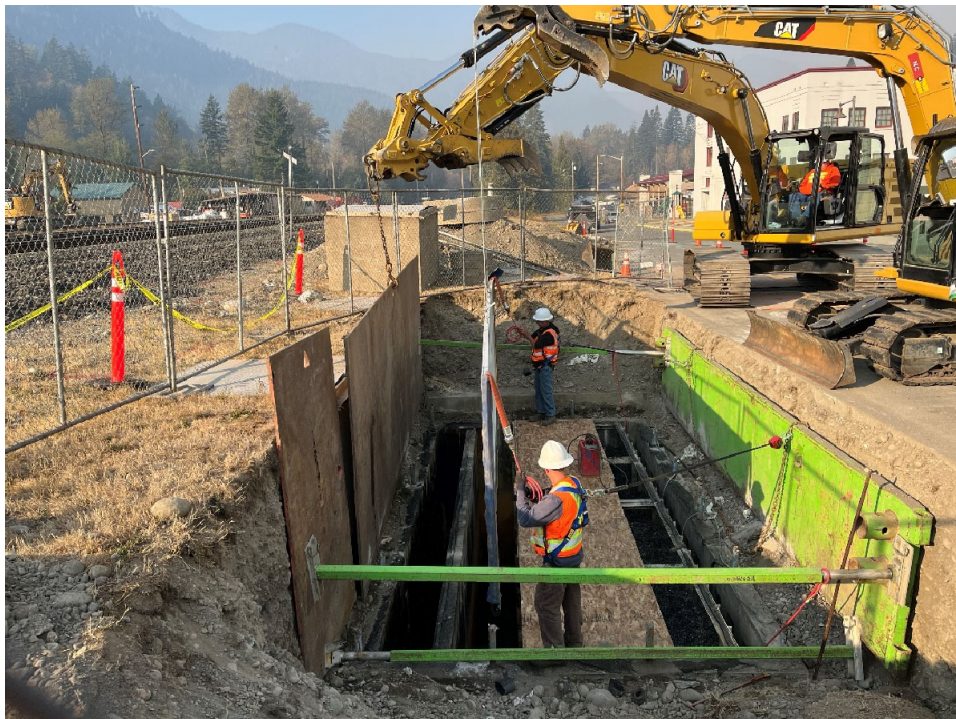
Photograph 10: Installation of Water Barriers.
