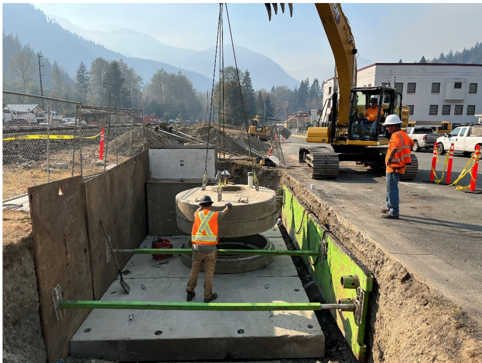
Photograph 20: Replacement of Risers.
