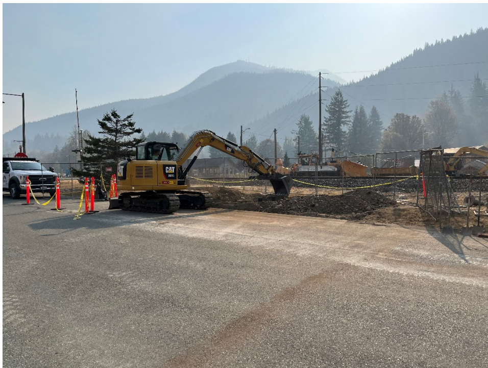
Photograph 26: Backfilling of Excavated Area.
