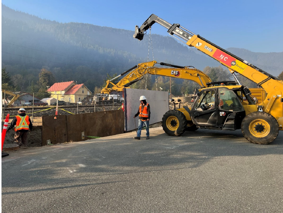
Photograph 9: Installation of Water Barriers.
