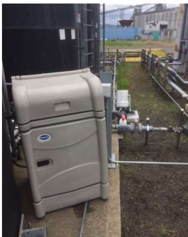
Figure 10.7: Automatic Sampler
