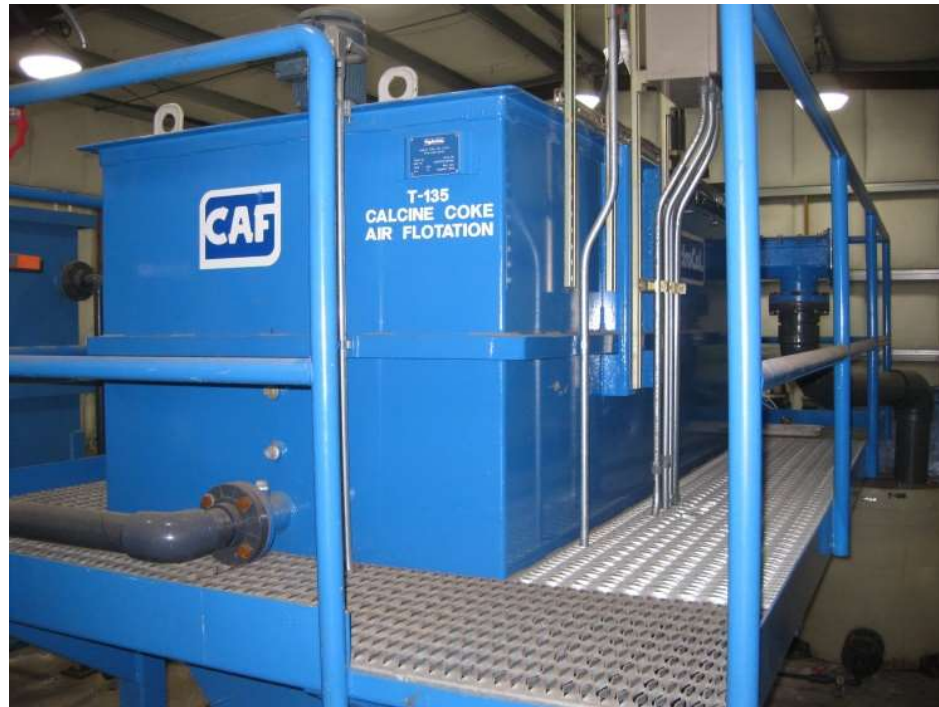
Figure 100.4: Cavitation Air Flotation Unit
