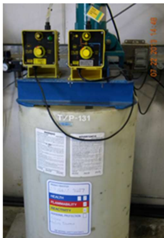
Figure 10.8: Polymer Tank T-131 and Chemical Metering Pumps
