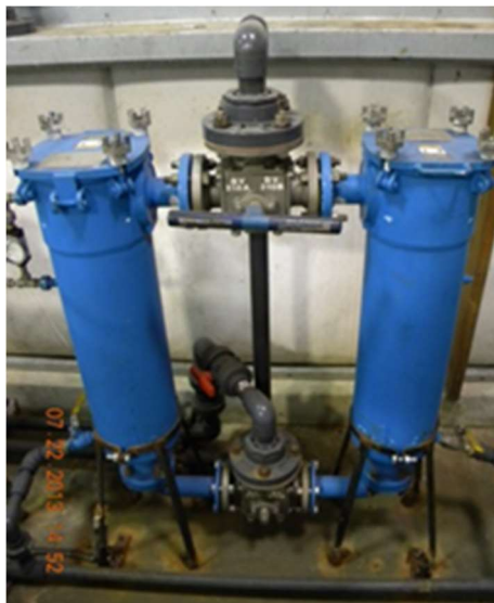
Figure 10.15: Bag Filtration System
