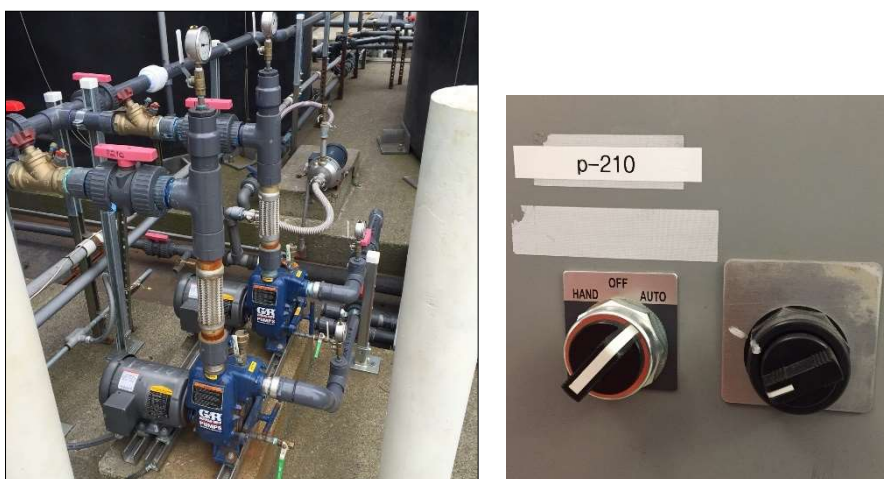
Figure 10.10: Pond Pumps P-210 & 220 and Control Knob for P-210
