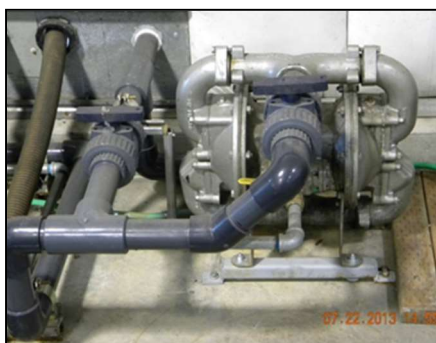
Figure 10.11: Sludge Pump P-125
