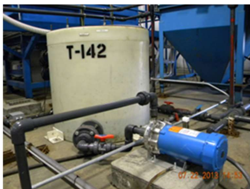
Figure 10.13: IPC T-140 Accepts Tank T-142 and Pump P-142
