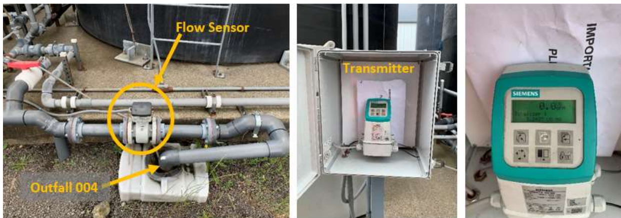
Figure 10.18: Discharge Flow Meter
