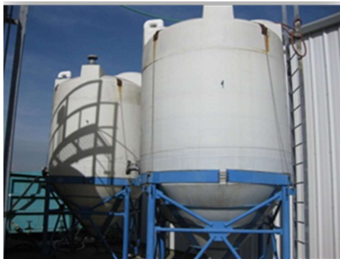
Figure 10.19: Sludge Holding Tanks
