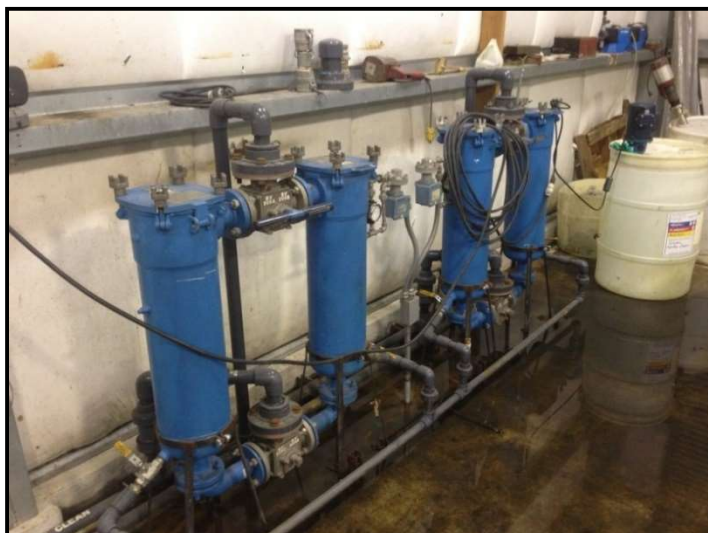
Figure 10.5: Duplex Bag Filters
