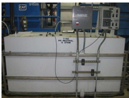
Figure 10.12: pH Neutralization Tank T-145
