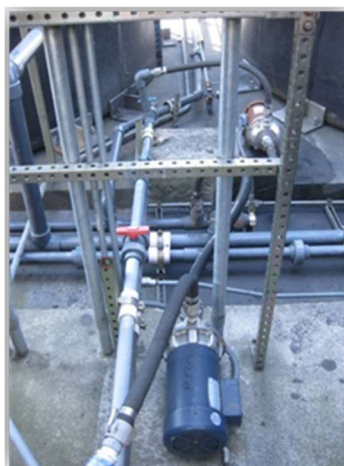
Figure 10.9: Transfer Pump
