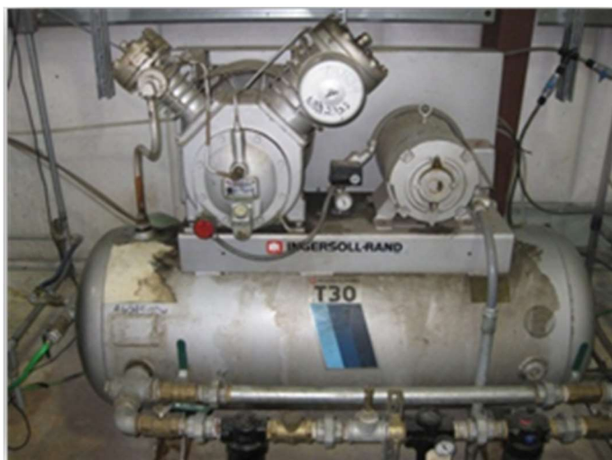
Figure 10.20: Air Compressor K-300
