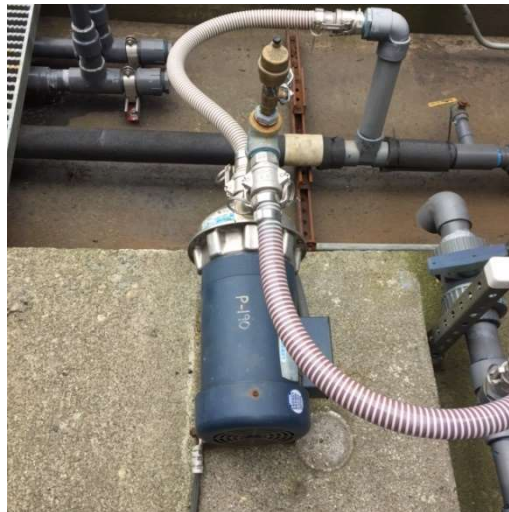
Figure 10.16: Effluent Pump P-190
