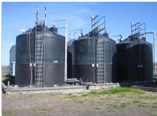
Figure 10.17: Clarified Water Storage Tanks T-170 and T-175
