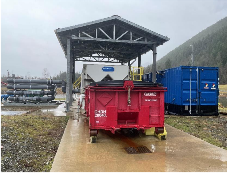
PHOTO #:05 DATE: 02/01/2024 TAKEN BY: JEANNE TRAN DESCRIPTION: ANOTHER VIEW OF THE DAF. THE RED COVER BIN STORES SLUDGE BUILDUP.
