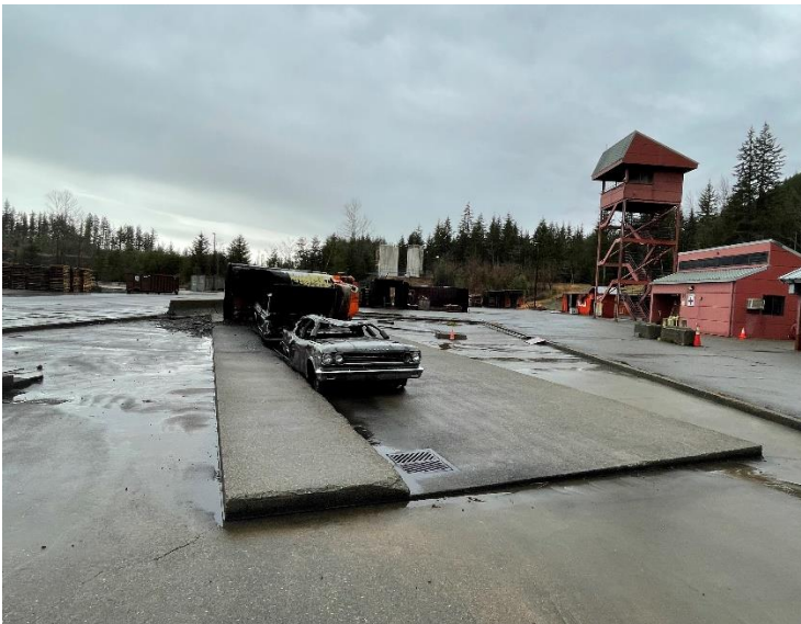
PHOTO #:15 DATE: 02/01/2024 TAKEN BY: JEANNE TRAN DESCRIPTION: ONE OF THE BURN PADS WITH PROP. NOTE THE DRAIN WITHIN THE BURN PAD TO COLLECT FIRE FIGHTING OILY WATER TO THE OIL WATER SEPARATOR.
