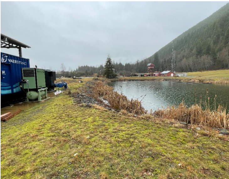
PHOTO #:07 DATE: 02/01/2024 TAKEN BY: JEANNE TRAN DESCRIPTION: THE TREATED WATER FROM THE DAF SYSTEM IS PUMPED TO POND 2 WHERE IT RECEIVES AERATION. SINCE THE DAF WAS BEING WINTERIZED, THE AERATION SYSTEM WAS NOT TURNED ON.
