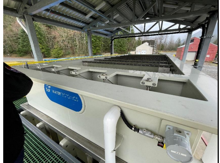
PHOTO #:06 DATE: 02/01/2024 TAKEN BY: JEANNE TRAN DESCRIPTION: THE TOP VIEW OF THE DAF UNIT. THE UNIT WAS BEING WINTERIZED AND NOT IN OPERATION DURING THE INSPECTION.
