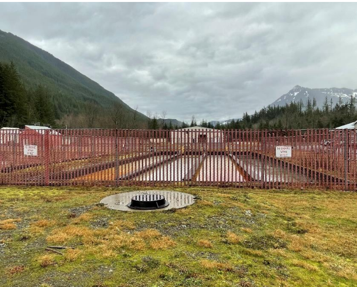
PHOTO #:19 DATE: 02/01/2024 TAKEN BY: JEANNE TRAN DESCRIPTION: OIL WATER SEPARATOR (OWS) WITH 5 BAYS. THE SKIMMER PUMP WAS NOT WORKING AND WAITING FOR REPAIR. THEY ARE ALSO WAITING FOR CLEAN HARBOR TO COME REMOVE THE WASTE OIL AND GET THE SEPARATOR BACK ONLINE.
