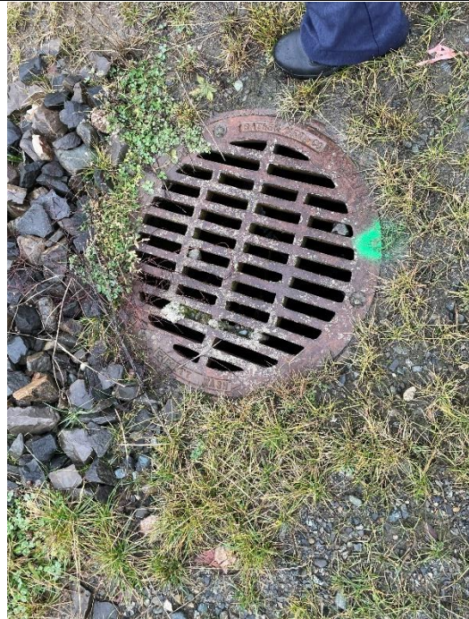
PHOTO #:24 DATE: 02/01/2024 TAKEN BY: JEANNE TRAN DESCRIPTION: ANOTHER DRAIN AND NO OILY SHEEN WAS OBSERVED AT THIS DRAIN EITHER.
