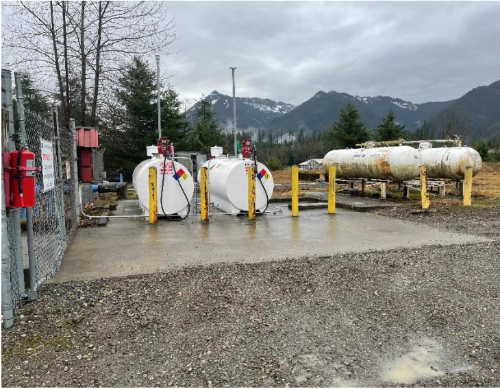
PHOTO #:13 DATE: 02/01/2024 TAKEN BY: JEANNE TRAN DESCRIPTION: A CLOSEUP VIEW OF THE HORIZONTAL DOUBLE-WALLED FUEL TANKS AND THE PROPANE TANKS.
