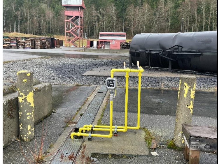
PHOTO #:18 DATE: 02/01/2024 TAKEN BY: JEANNE TRAN DESCRIPTION: FUEL METER TO MEASURE THE AMOUNT OF FUEL USED AT BURN PAD FOR EACH FIREFIGHTING EXERCISE.
