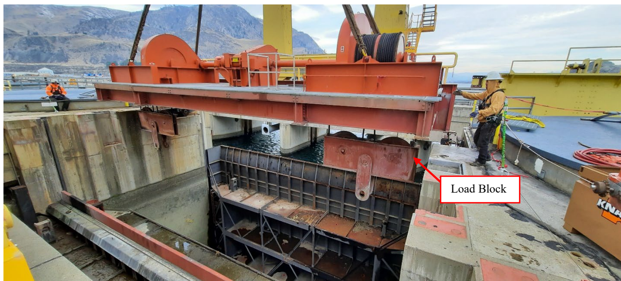
Figure 4 Wells Project Spillway Hoist Being Lifted Out of a Spillway
