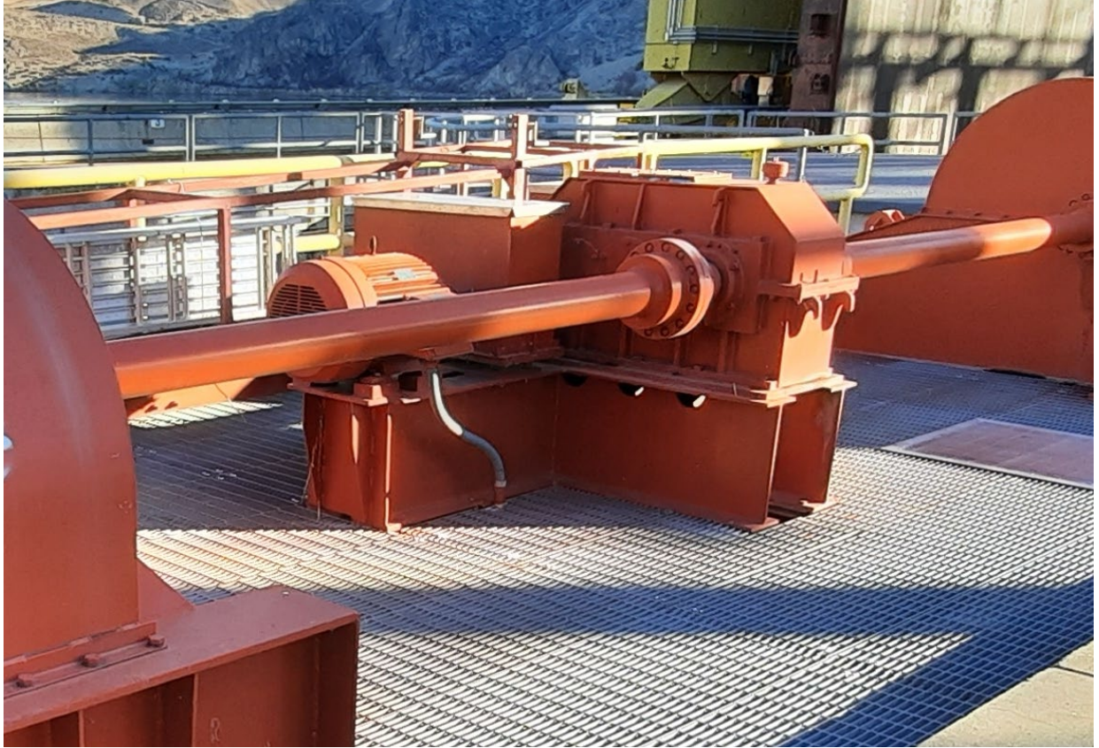
Figure 17. Wells Project Spillway Hoists Gear Reducing Gearbox
