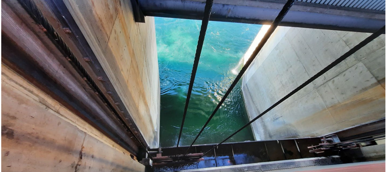
Figure 5 Wells Project Lower Leaf Vertical Leaf Gate Connected to Gate Hoist with Wire Rope
