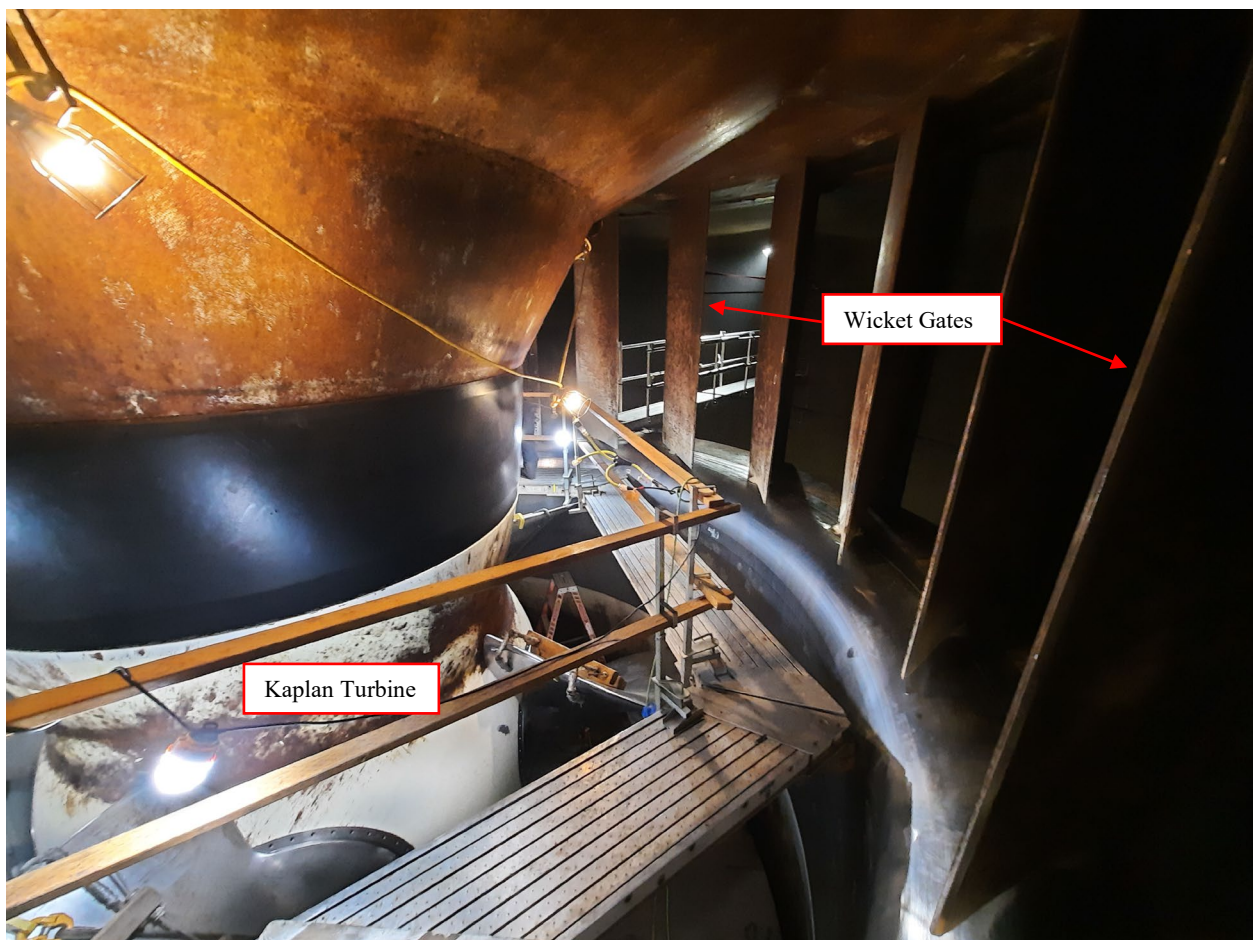
Figure 8. Wells Project Wicket Gates shown with Turbine Assembly Installed
