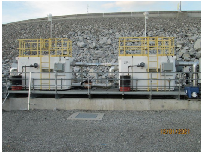
Figure 2. Oil Water Separator (Outfall No. 2)
