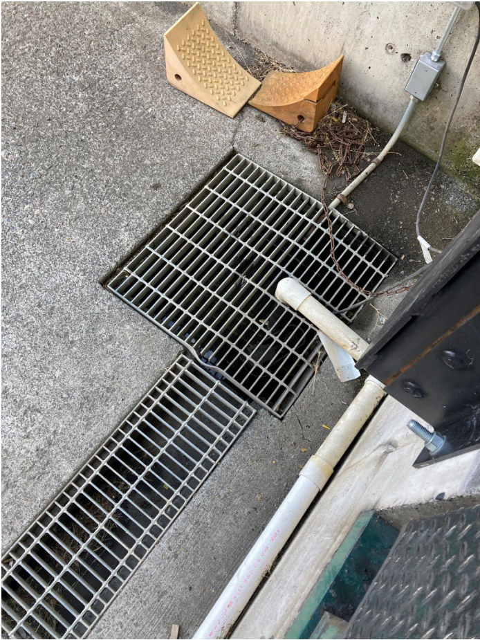
Photo 2 [IMG_0538] Description: Stormwater sump – all floor drains from inside the warehouse go here
