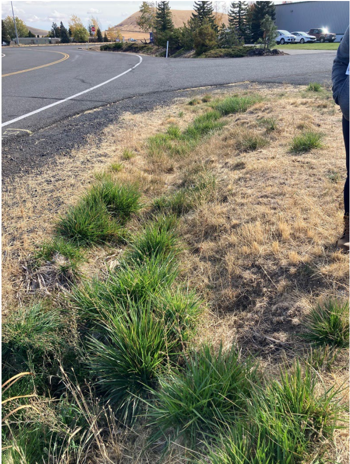
Photo 3 [IMG_0539] Description: Stormwater ditch where sump is discharged when valve is turned on
