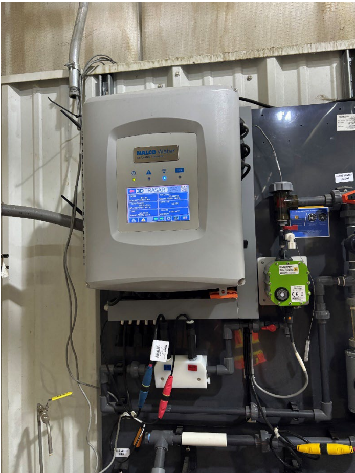
Photo [10] [IMG_3612] Description: Blowdown Water Monitoring Panel
