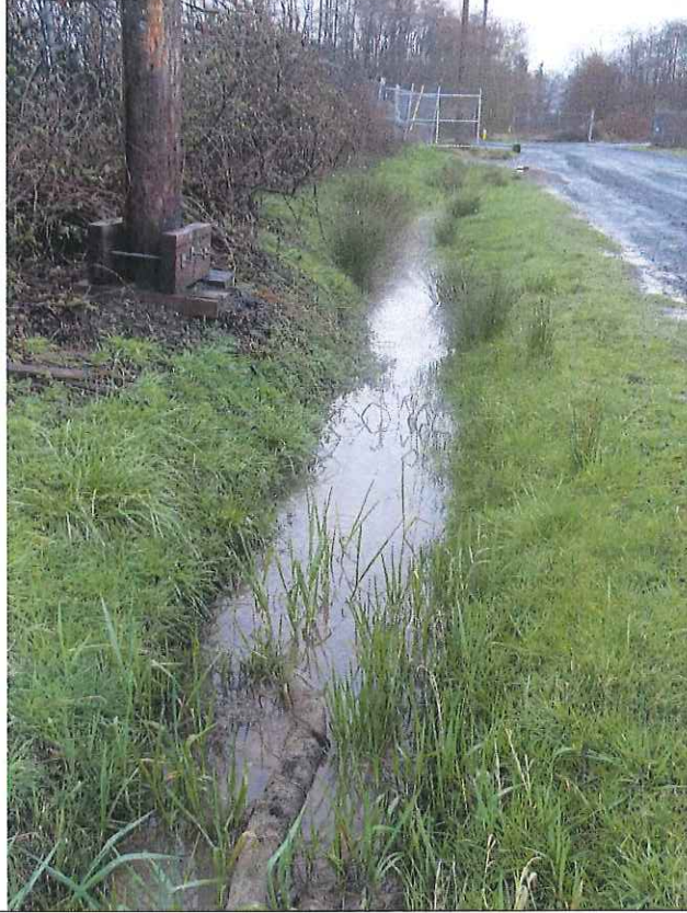
Photo 9 of 12: Ditch leaving the site to Grays Harbor had oil and high turbidity. Site not maintaining BMPs.
