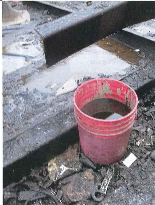
Photo 8 of 12: Open oil containers stored outside, no secondary containment and exposed to stormwater.
