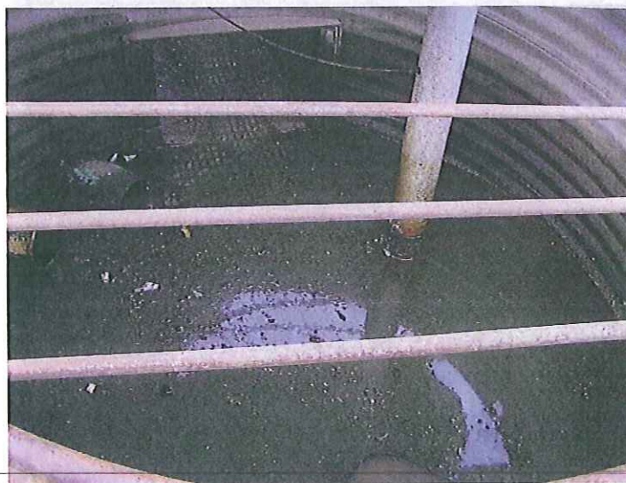
PHOTO #:12 DATE: 11/04/2010 TAKEN BY: : LORI LEVANDER DESCRIPTION: TANK WHERE FLOCCULATION AGENT IS ADDED TO WASHWATER PRIOR TO ENTERING POND #1.
