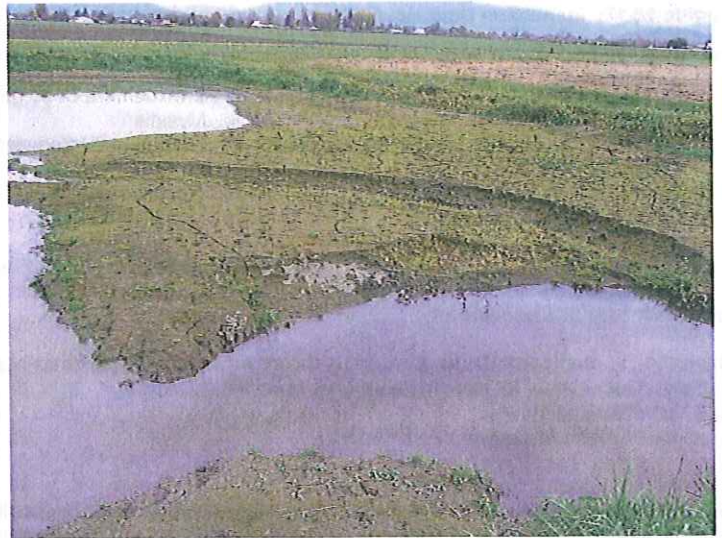
PHOTO #:02 DATE: 11/04/2010 TAKEN BY: LORI LEVANDER DESCRIPTION: SOLIDS BUILD-UP AT HEAD END OF POND #1. DRIED UP POND (NO LONGER USED) IN BACKGROUND.
