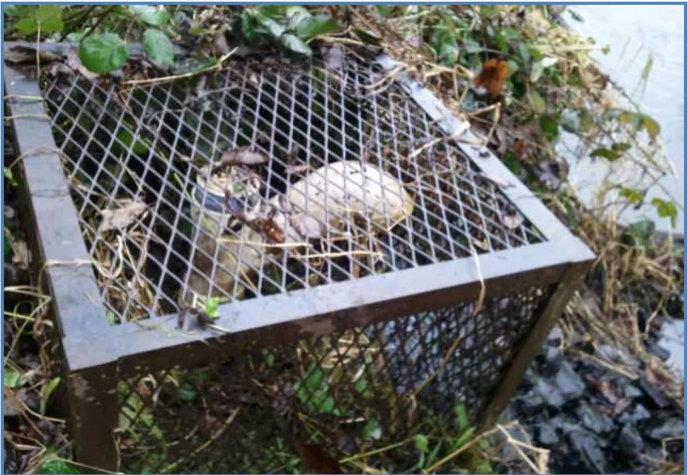
**Photograph Note:** Photo of the outfall during the inspection. Note that vegetation has been removed and structures is clear and draining normally (out to the right of the photo).
