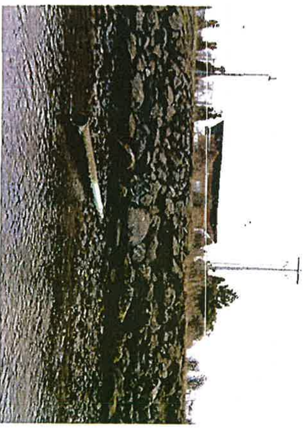
Photo 2 – Closer view of existing storm drain outfall on beach to be removed. Pump Station 4 (to be demolished) directly above. Feb 11, 2014.
