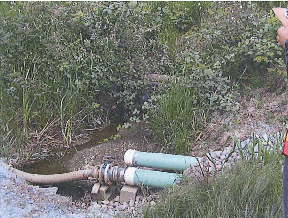
PHOTO #:09 DATE: 06/09/14 TAKEN BY: JEANNE TRAN DESCRIPTION: HUGHES FARMS PIPED THE WATER FROM THE SETTLING POND TO THE FARM FIELD LOCATED ACROSS THE STREET FROM THEIR PLANT.
