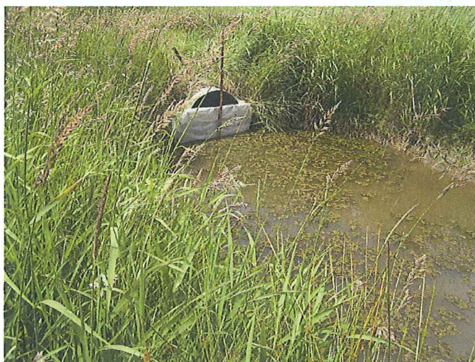
PHOTO #:22 DATE: 06/09/14 TAKEN BY: JEANNE TRAN DESCRIPTION: A MAN-MADE PLYWOOD COVERED WITH PLASTIC TO ISOLATE THE WATER IN THE FIELD DITCH.
