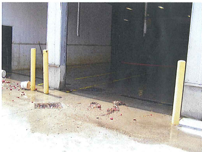
PHOTO #:23 DATE: 06/09/14 TAKEN BY: JEANNE TRAN DESCRIPTION: A VIEW AT THE POTATO OFF-LOADING AREA. FLOOR WASH WATER IS DRAINED TO THE UNDERGROUND VAULT.
