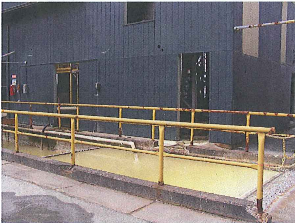
PHOTO #: 03 DATE: 06/09/14 TAKEN BY: JEANNE TRAN DESCRIPTION: A VIEW OF THE CONCRETE TROUGH LOCATED IN THE BACK OF CHEMTRADE SULEX'S PLANT. THIS TROUGH IS USED FOR COLLECTING PRILLED SULFUR CONTACT WATER FOR REUSE.
