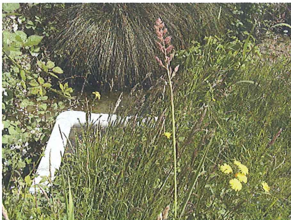
PHOTO #:11 DATE: 06/09/14 TAKEN BY: JEANNE TRAN DESCRIPTION: A VIEW OF THE PVC PIPE TRANSPORTING THE WATER TO THE FARM FIELD. THE PVC PIPE RUNS UNDERNEATH THE ROAD, ACROSS THE STREET TO THE FARM FIELD.
