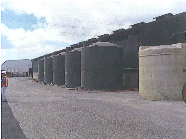
PHOTO #: 05 DATE: 06/09/14 TAKEN BY: JEANNE TRAN DESCRIPTION: SIX NEW STORAGE TANKS WERE RECENTLY INSTALLED TO HOLD ALL WATER COLLECTED FROM THE SITE, INCLUDING STORMWATER, FOR REUSE PURPOSES.
