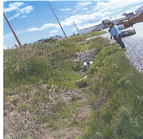
PHOTO #:10 DATE: 06/09/14 TAKEN BY: JEANNE TRAN DESCRIPTION: ANOTHER VIEW OF THE SETTLING POND'S OUTLET PIPE CONNECTING TO A HOSE WHICH CARRIES THE WATER TO THE FARM FIELD.
