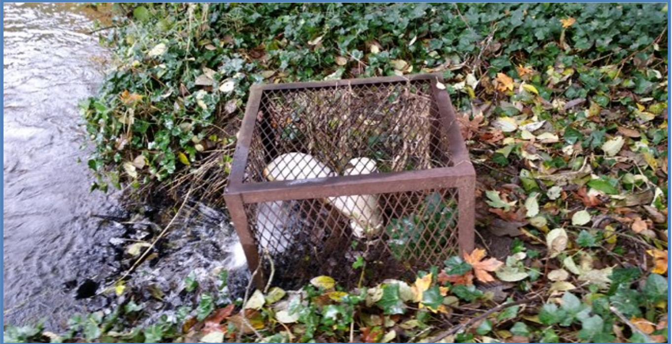
**Photograph Note:** Photo of the outfall during the inspection. The outfall structure is clean and draining normally (drainage is toward the left into Burnt Bridge Creek).
