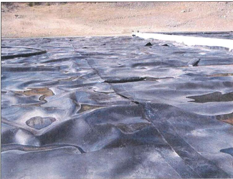
An aerial photograph showing a large, rectangular concrete basin. The interior of the basin is covered with a dark, wrinkled material, identified as HDPE liner. The surrounding area is a dry, hilly landscape with sparse vegetation.                                                     |
