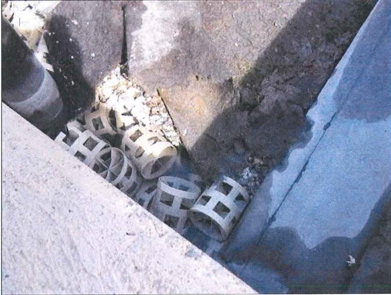
A close-up photograph showing white, lattice-like plastic media (likely Kaldnes K1) installed in a concrete-lined biotreatment tank. The media is partially submerged in water, and a pipe is visible on the left side of the frame.               |
