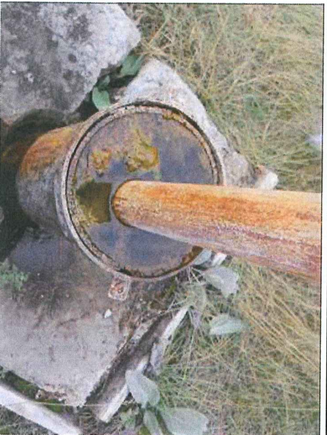
LF-4 (artesian) well and standpipe.
