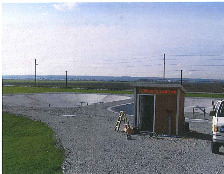
PHOTO #:06 DATE: 11/04/15 TAKEN BY: JEANNE TRAN DESCRIPTION: PICTURE SHOWS TWO NEWLY CONSTRUCTED LINED PONDS, AND AN EQUIPMENT CONTROL SHED.
