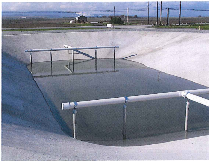
PHOTO #:08 DATE: 11/04/15 TAKEN BY: JEANNE TRAN DESCRIPTION: WASHWATER WILL ENTER THE PRIMARY SETTLING POND THROUGH THE PERFORATED PIPE. FLOCCULENT AGENT WILL BE INTRODUCED INTO THE INCOMING LINE BEFORE ENTERING THE POND.
