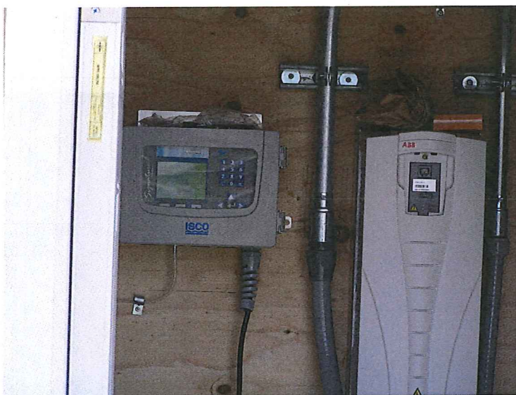
PHOTO #:07 DATE: 11/04/15 TAKEN BY: JEANNE TRAN DESCRIPTION: CONTROL PANEL FOR FLOW AND PH METERS IN THE SHED.
