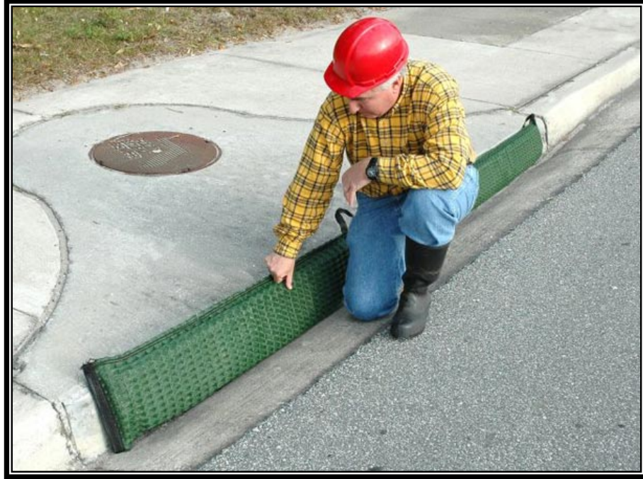
Figure 4.20. Commercially Available Gutter Guard Being Replaced.
