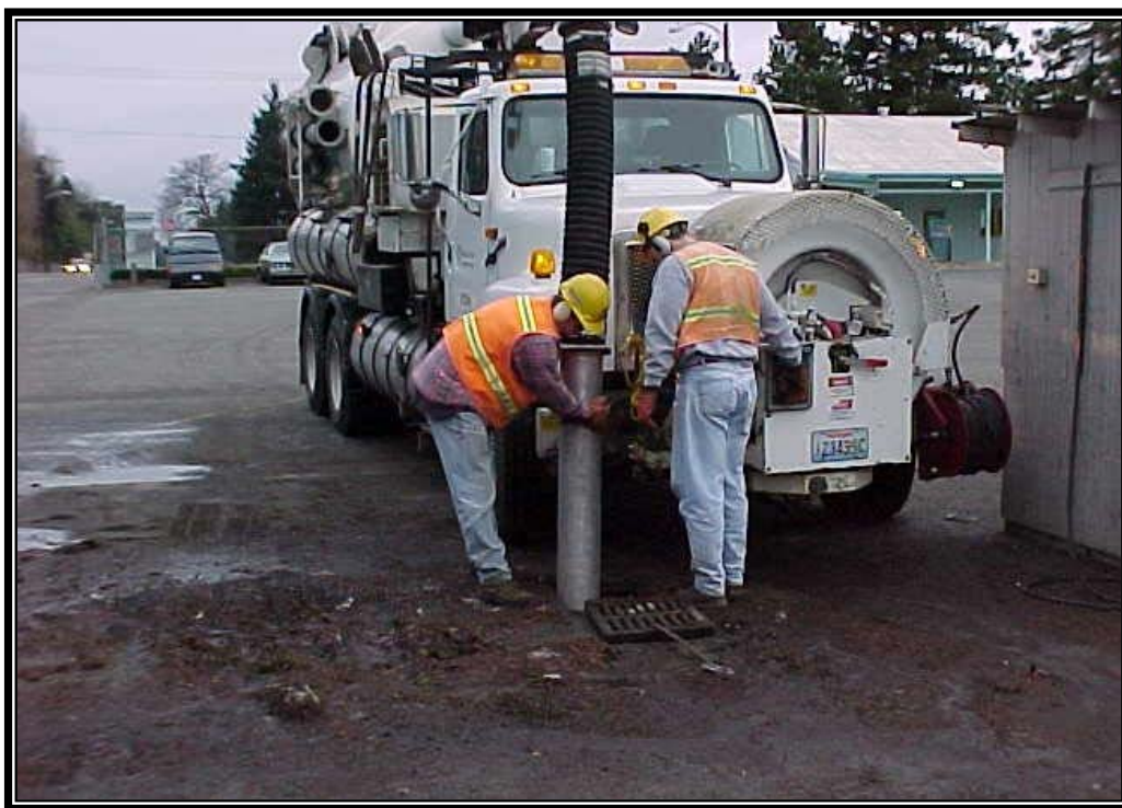
Figure 4.23. Catch Basin Cleaning with a Vacuum Truck.
