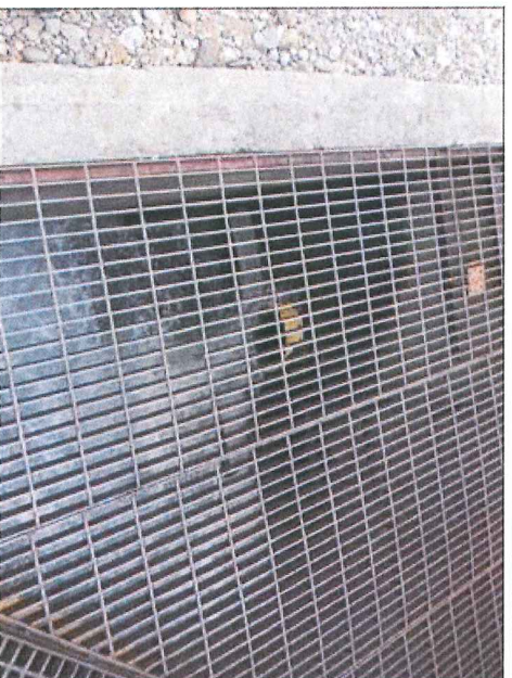
Downstream of internal north outfall (outfall 004) flume structure. Settled backwash from the effluent black walnut shell filters discharges here, along with treated sanitary and industrial process wastewaters.
