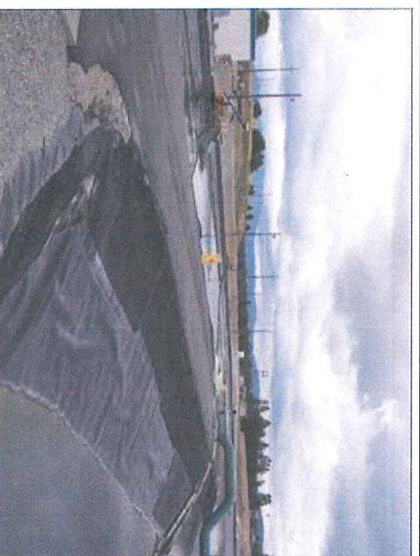
Effluent weir of secondary clarifier at sanitary wastewater treatment plant.
