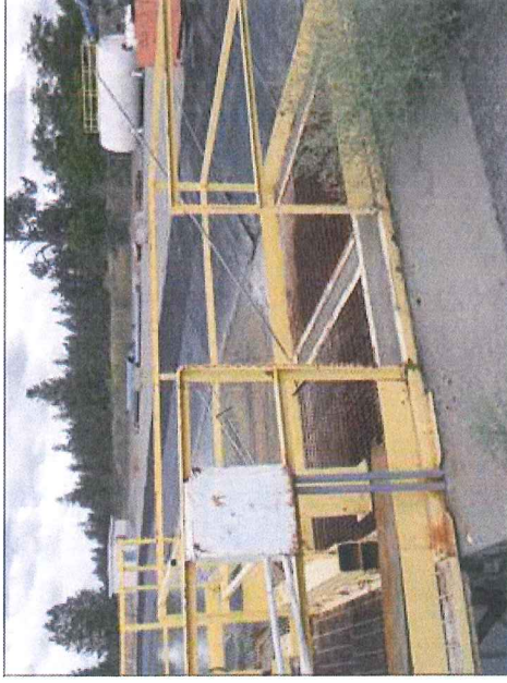
Outlet of wastewater settling lagoon. Plant personnel remove oil accumulated on the surface via a pumper truck.
