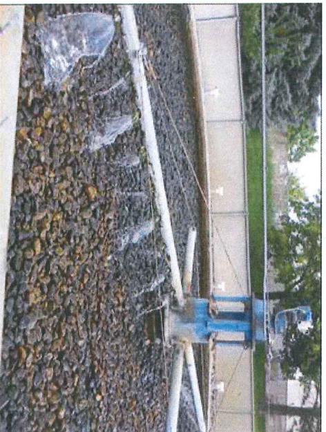
Trickling filter at sanitary wastewater treatment plant.
