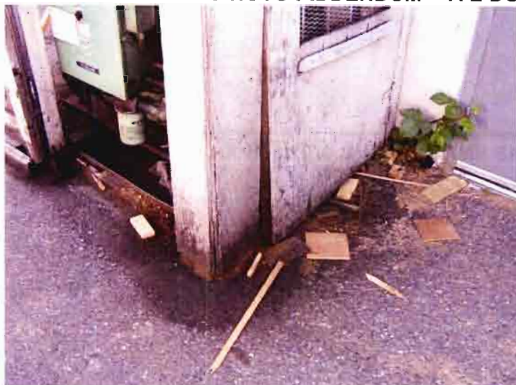
P5160035 DESCRIPTION: OIL LEAKING OUT AROUND COMPRESSOR SHED
