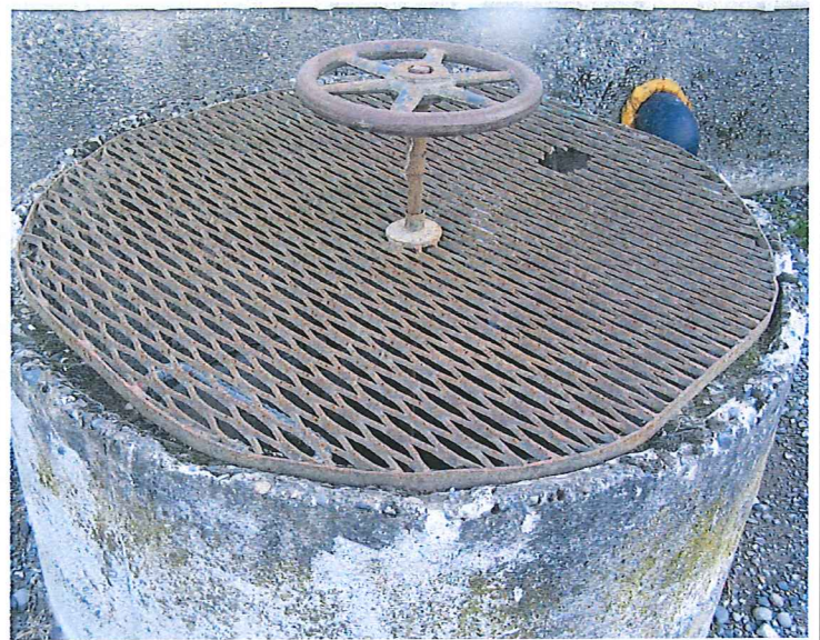
PHOTO #02 DATE: 09/08/16 TAKEN BY: JEANNE TRAN DESCRIPTION: A CLOSED UP PICTURE OF THE UNDERGROUND SUMP, WHICH HAS A MANUAL VALVE TO CONTROL THE DISCHARGE TO THE PONDS.
