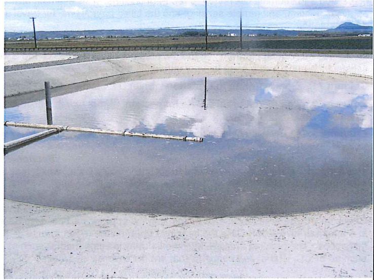
PHOTO #04 DATE: 09/08/16 TAKEN BY: JEANNE TRAN DESCRIPTION: A CLOSED UP PICTURE OF THE FIRST POND. EACH POND IS DESIGNED TO HANDLE A FLOW RATE OF 130 GPM WITH 13 HOUR SETTLING TIME AFTER DOSING WITH A FLOCCULATING AGENT TO AID IN THE SEDIMENTATION OF THE WASTEWATER.
