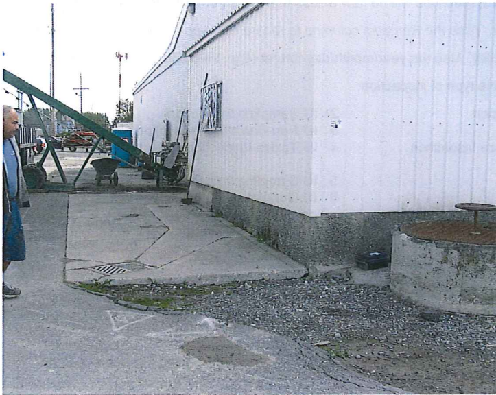
PHOTO #01 DATE: 09/08/16 TAKEN BY: JEANNE TRAN DESCRIPTION: PICTURE SHOWS AN UNDERGROUND COLLECTION SUMP FOR THE PLANT. THIS SUMP HAS BEEN PLUMBED TO DRAIN TO THE TWO NEWLY CONSTRUCTED LINED PONDS FOR TREATMENT.
