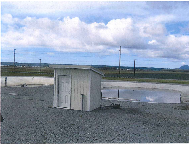
PHOTO #03 DATE: 09/08/16 TAKEN BY: JEANNE TRAN DESCRIPTION: A VIEW OF THE TWO NEWLY CONSTRUCTED LINED PONDS CONNECTED IN SERIES. ONE SERVES AS A PRIMARY POND, THE SECOND SERVES AS THE SECONDARY POND TO POLISH THE TREATED WATER FROM THE FIRST POND.
