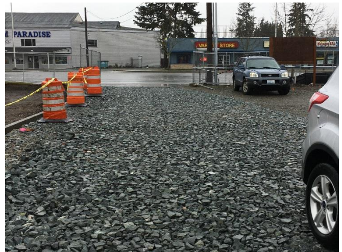
STABILIZED CONSTRUCTION ACCESS
