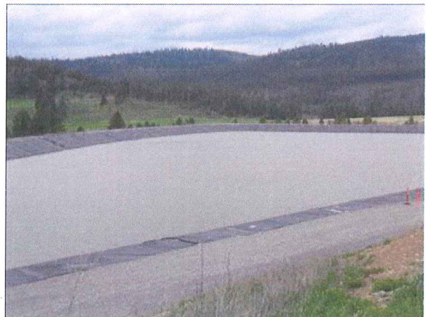
The lined groundwater management impoundment. The liner system consists of two liners with a leak recovery collection system.
