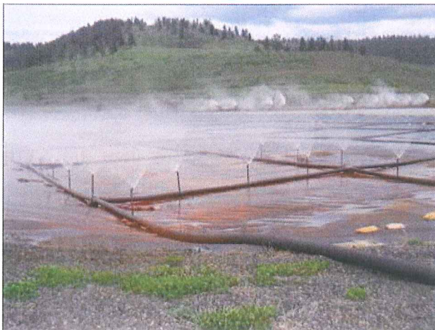
The lined enhanced evaporation area adjacent to the groundwater management impoundment. Water from this area drains back into the groundwater management impoundment.
