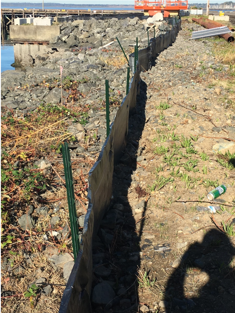
Photo 3 – Wire backed silt fence.
