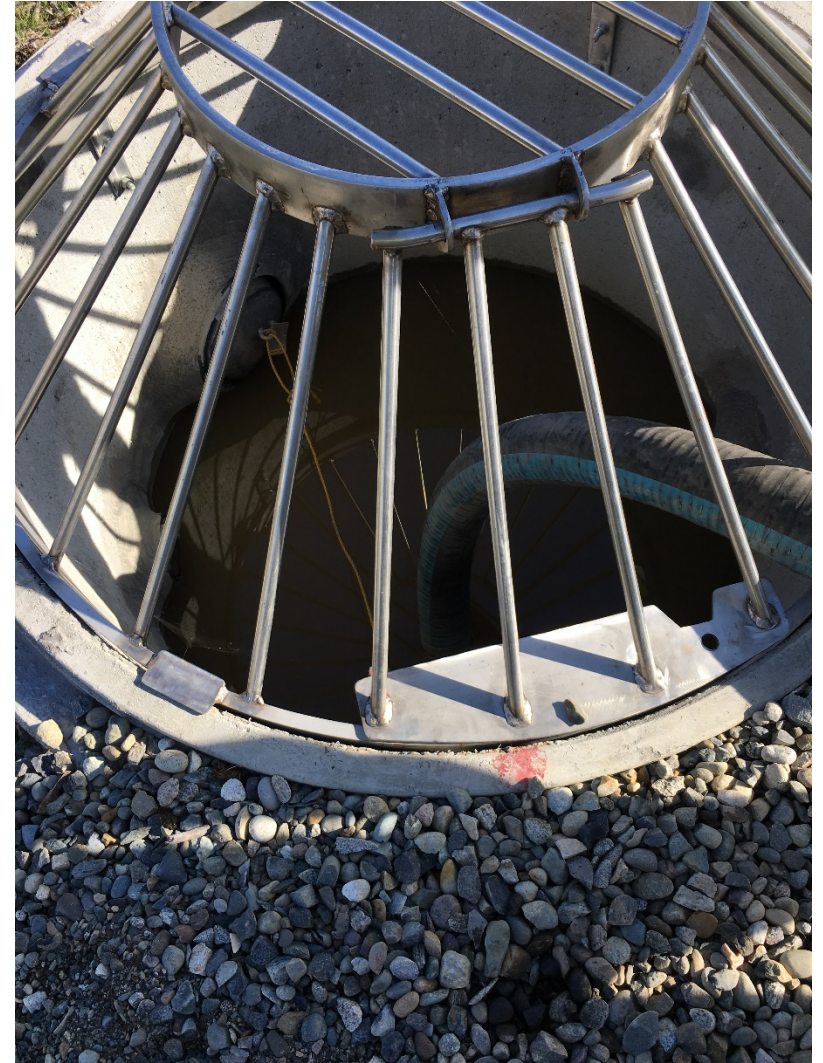
Photo 2 – Plugged outlet and hose for pump at existing MFD form phase 1
