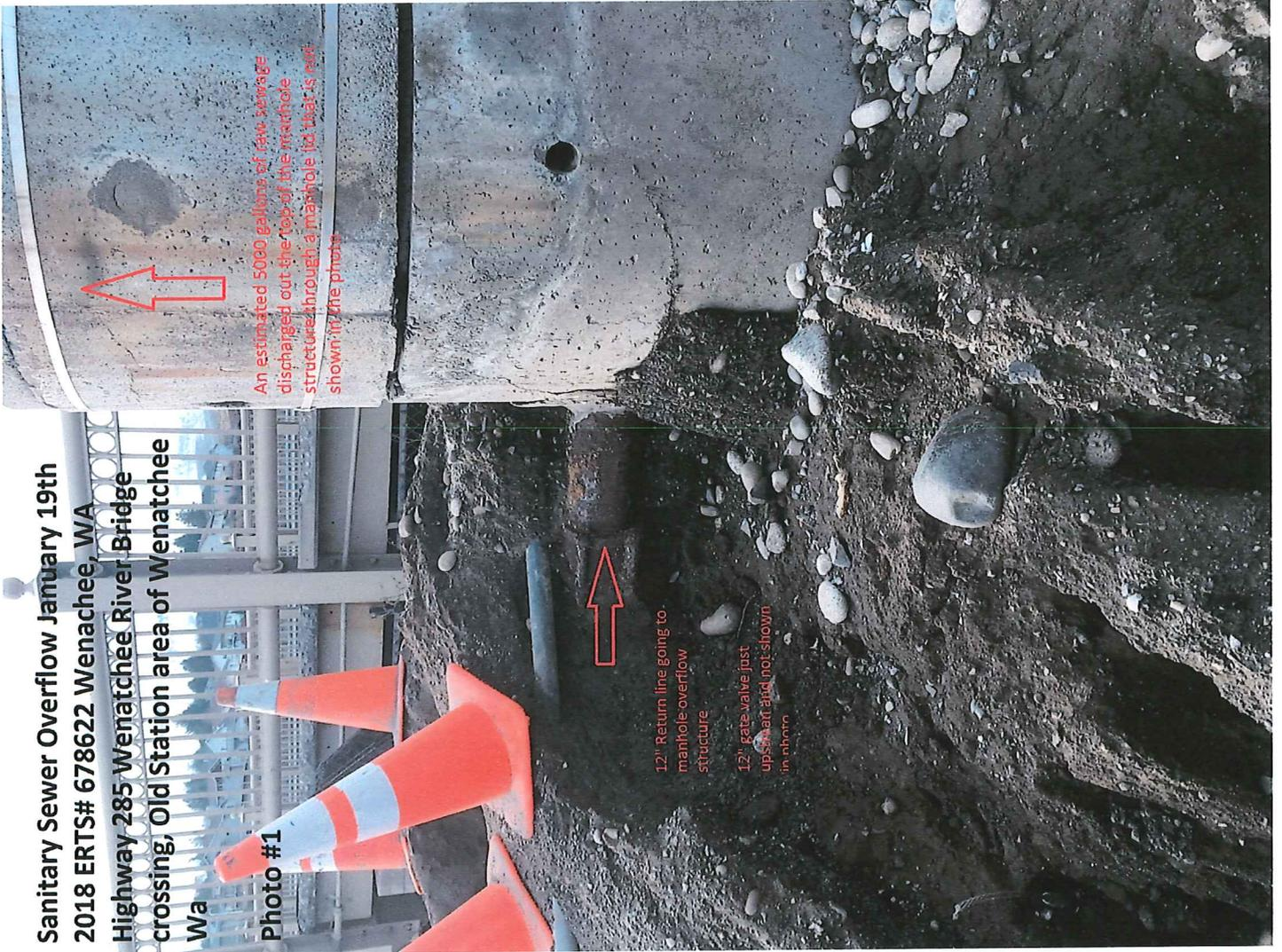
An estimated 5000 gallons of raw sewage discharged out the top of the manhole structure through a manhole lid that is not shown in the photo
