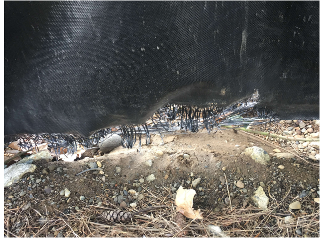
DESCRIPTION: SILT FENCE THAT IS NO LONGER TRENCHED IN.
