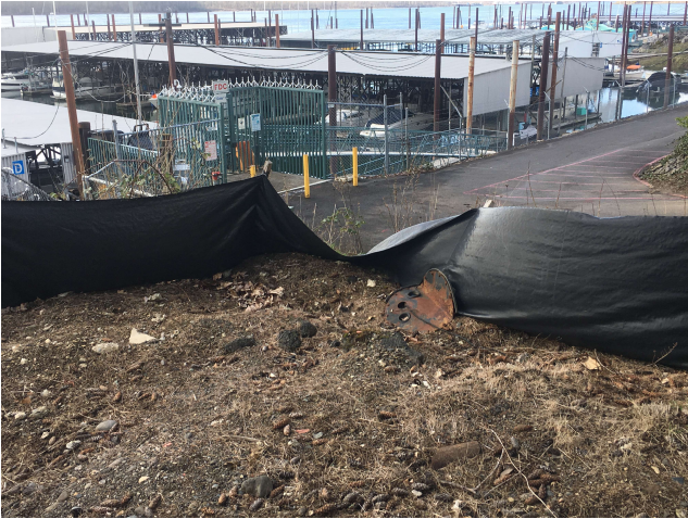
DESCRIPTION: SILT FENCE IN NEED OF MAINTENANCE.
