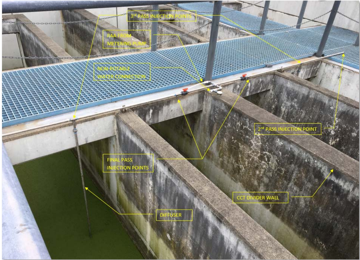
FIGURE 2-4: PAA INJECTION LOCATIONS IN THE CCT
