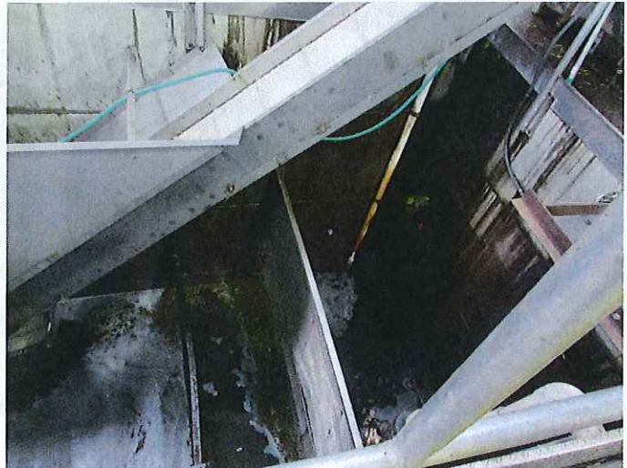
Sump pit that includes screens to evaporative lagoon
