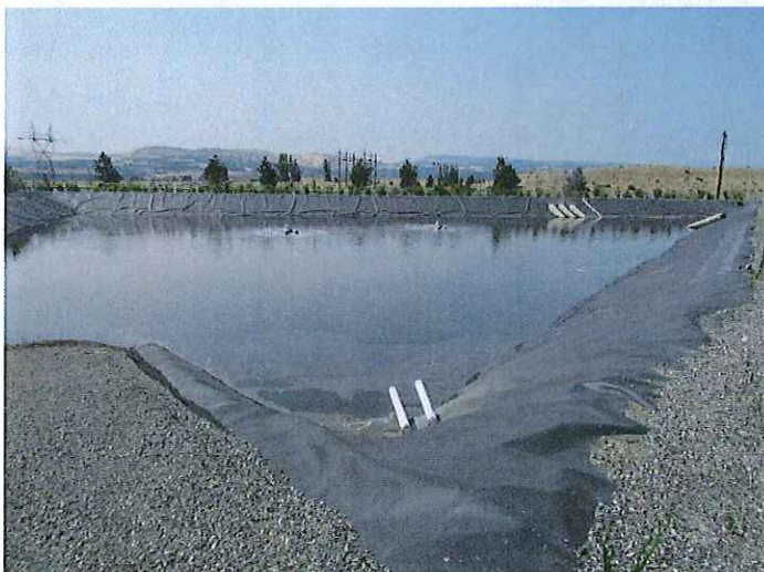
Lined evaporative lagoon (in let pipes foreground; outlet to POTW background).
