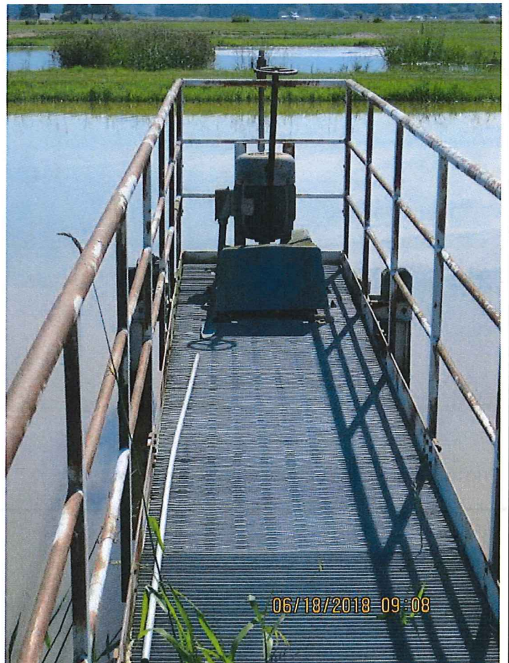
PHOTO 20 DESCRIPTION: RECYCLE PUMP FOR WATER REUSE IN PLANT OPERATIONS.
