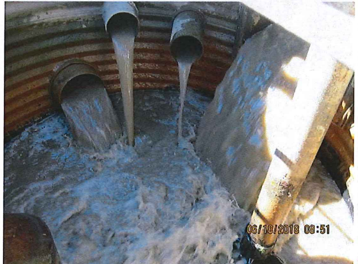
PHOTO 4 DESCRIPTION: DISCHARGES FROM ROTARY WASHER AND FLOOR DRAINS.
