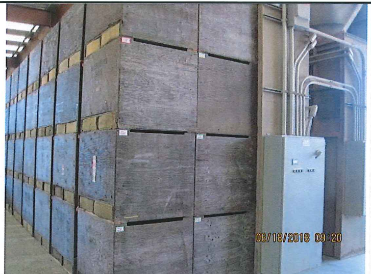
PHOTO 22 DESCRIPTION: CRATES OF WASHED BULBS BEING AIR DRIED. AIR PLENUM IS BEHIND CONTROL BOX. BOXES HAVE SCREENED BOTTOMS. AIR MOVES UP THROUGH BOXES AND EXIT THROUGH OPENINGS ON THE ENDS.
