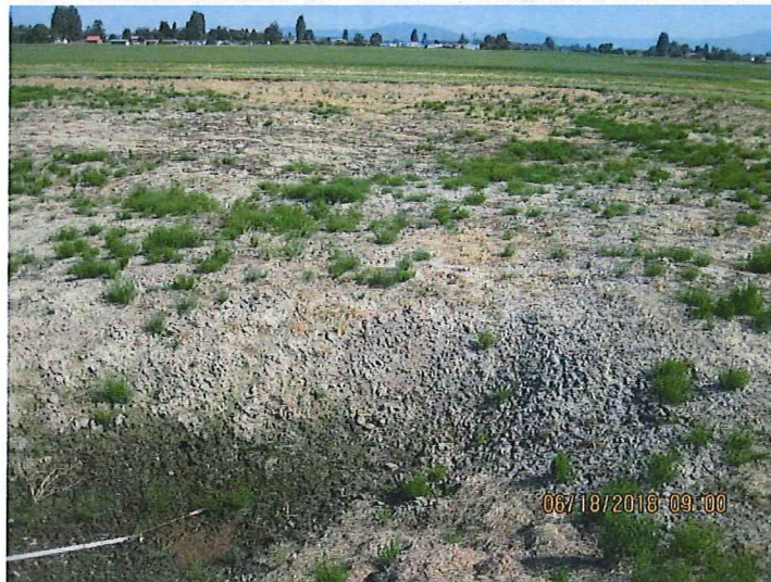
PHOTO 14 DESCRIPTION: SETTLING POND 1, FULL OF SEDIMENT.
