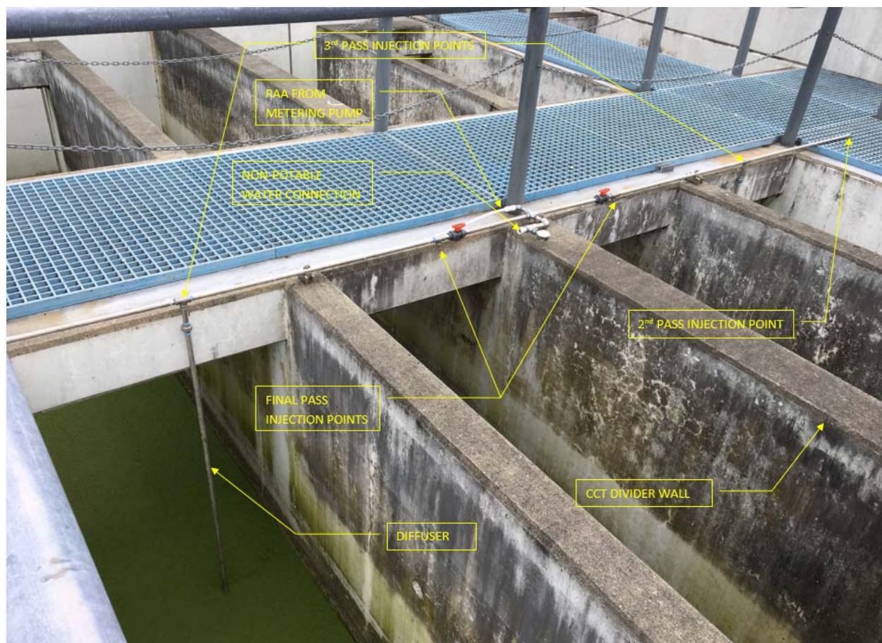
FIGURE 2-4: PAA INJECTION LOCATIONS IN THE CCT
