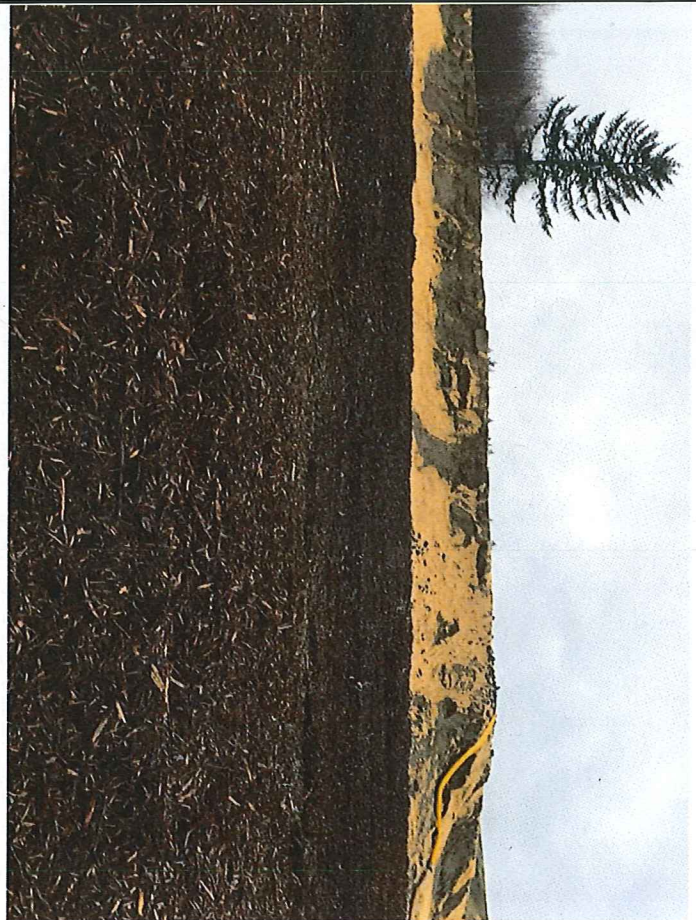
02 DESCRIPTION: SLUFFING ON OUTSIDE WALLS OF LOWER POND SHOWS SIGNS OF POTENTIAL FAILURE.
