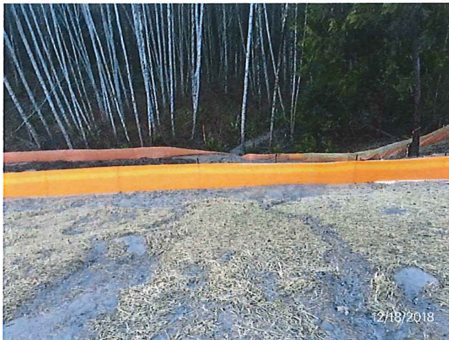
03 DESCRIPTION: DISCHARGE OF STORMWATER AND SEDIMENT INTO WETLAND BELOW 1 ST POND.
