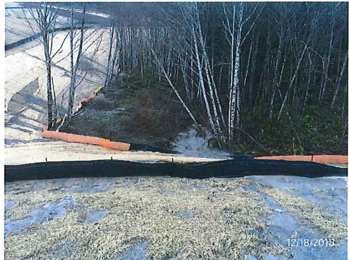
04 DESCRIPTION: DISCHARGE OF STORMWATER AND SEDIMENT IN MANY LOCATIONS INTO ADJACENT WETLANDS.
