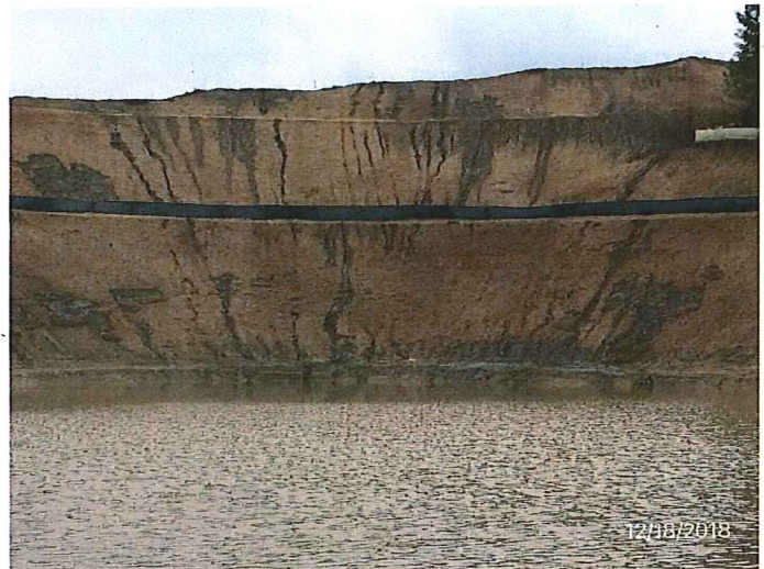
12 DESCRIPTION: LARGE AMOUNT OF RILLING ON HILLSIDE AND INADEQUATE SLOPE BMPs.
