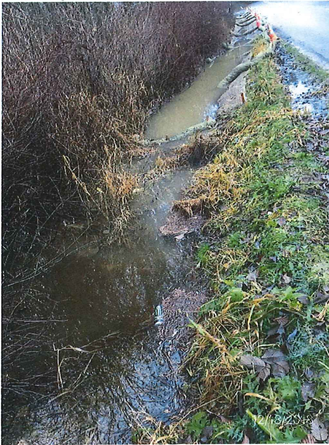
09 DESCRIPTION: PHOTO OF DISCHARGE FROM SITE ONTO GLENWOOD RD INTO RUBY CREEK TRIBUTARY.
