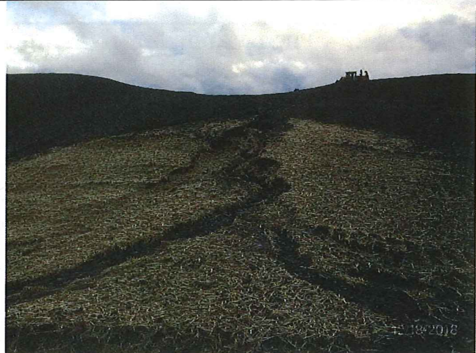
06 DESCRIPTION: HEAVY RILLING ON SLOPES ALONG BACKSIDE OF PROJECT. INADEQUATE SLOPE BMPs OR NO BMPs PRESENT.
