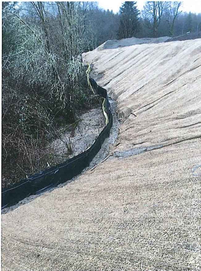
01 DESCRIPTION: DISCHARGE OFFSITE OF STORMWATER AND SEDIMENT VIA OVERTOPPING SILT FENCING INTO WETLANDS.
