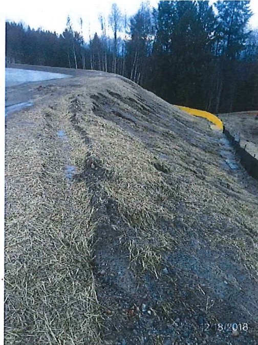
02 DESCRIPTION: 1 ST POND SE SIDE SHOWING SIGNS OF SOIL SATURATION AND SLUFFING ISSUES.
