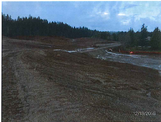
05 DESCRIPTION: BACKSIDE OF PROJECT STILL COMPLETELY BARE SOIL WITH NEW ROADWAY AND POND BEING FILLED FROM LOWER PONDS.
