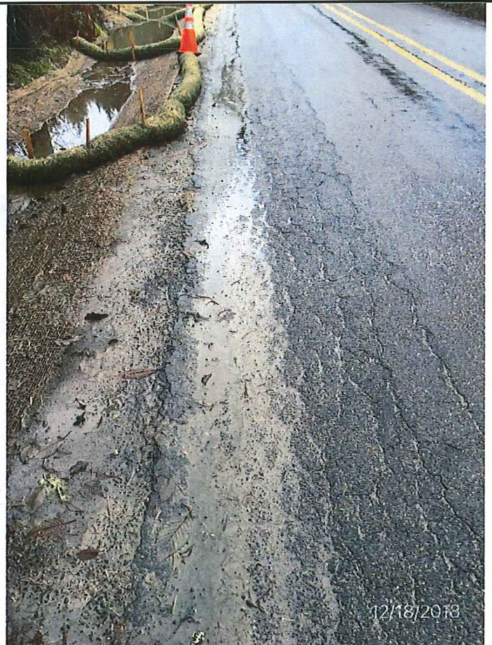
10 DESCRIPTION: SEDIMENT PRESENT ON ROADWAY SHOWING SIGNS OF LARGER DISCHARGE RECENTLY.
