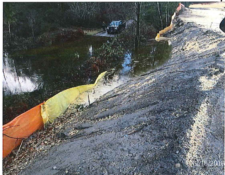
08 DESCRIPTION: FRONT OF SITE HAS CAUSED FLOODING ON NEIGHBORS PROPERTY. DRIVEWAY INACCESSIBLE WITH PICKUP TRUCK.
