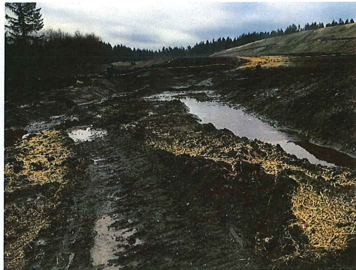
Photo 6 Description: The channels to pond between the two eastern ponds have rock check dams, but are not lined.
