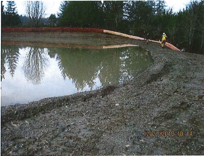
Photo 1 Description: Pond in the Northwest corner of site is full. Soils around pond are bare.
