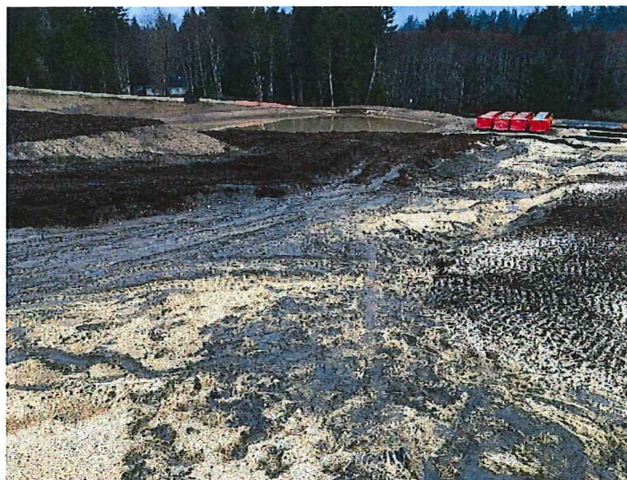
Photo 8 Description: Northeast pond level is several feet below the top of the pond. There are four baker tanks beside it.
