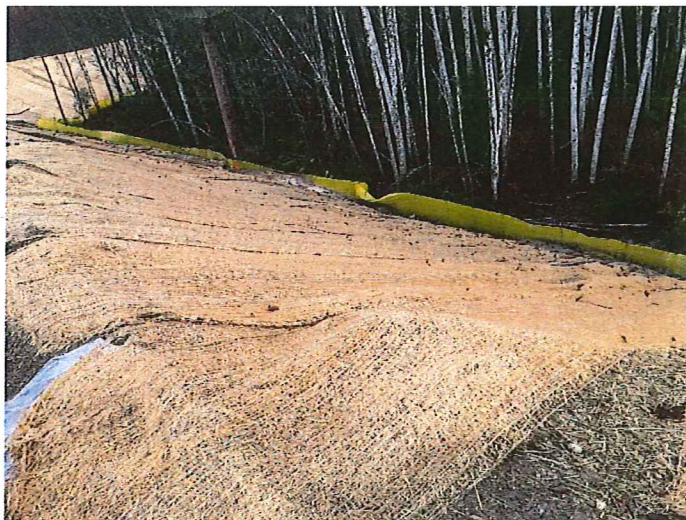
Photo 9 Description: Silt fence around wetland needs maintenance.
