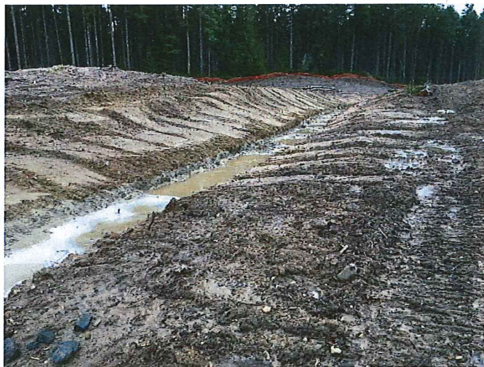
Photo 5 Description: Channel to western pond is not lined.
