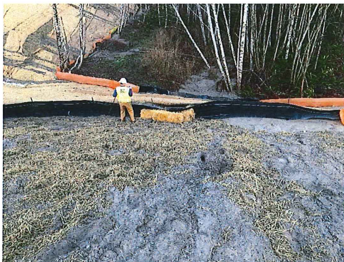
Photo 11 Description: Slope above wetland needs to be stabilized.
