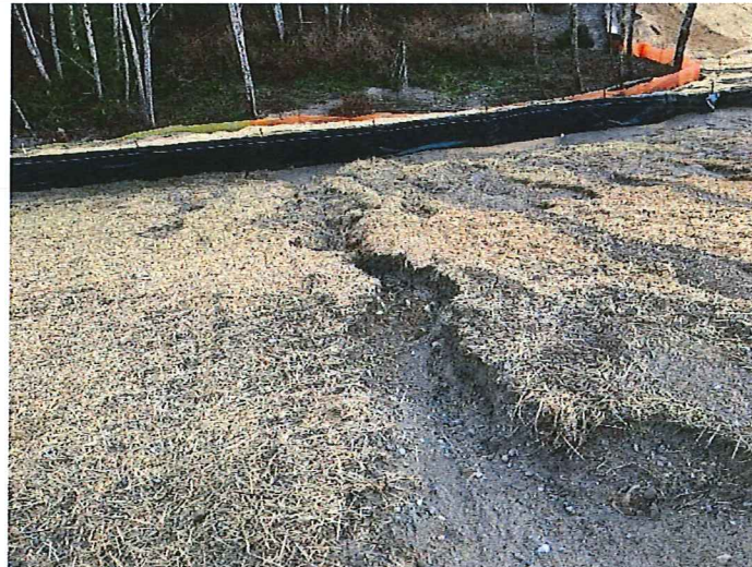
Photo 10 Description: Slope above wetland needs to be stabilized.
