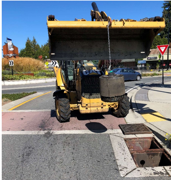
City Maintenance Crews replace cartridge filters at a public water quality facility.
