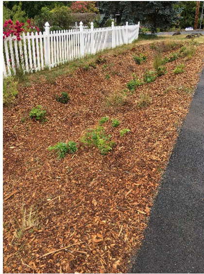
The City continues to seek opportunities for LID retro-fit; including this newly install bio-retention area.
