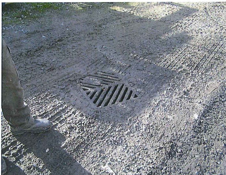
PHOTO #:13 DATE: 01/16/19 TAKEN BY: JEANNE TRAN DESCRIPTION: A CLOSE UP PICTURE OF THE NEARBY STORM DRAIN MENTIONED IN PHOTO# 12. THIS DRAIN WAS PLUGGED WITH SEDIMENT, AND THE AREA WAS MUDDY AS CAN BE SEEN ON THE PHOTO. ACCORDING TO JOSE, THIS DRAIN IS CONNECTED TO THE LAGOONS.
