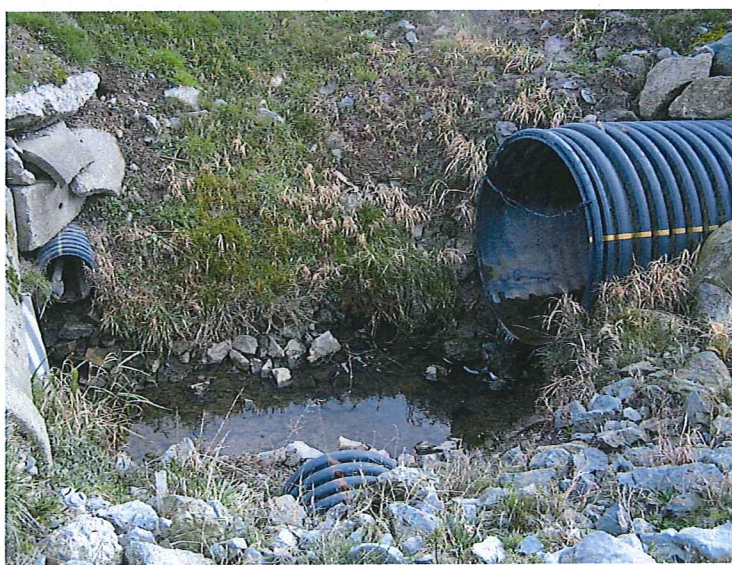
PHOTO #:20 DATE: 01/16/19 TAKEN BY: JEANNE TRAN DESCRIPTION: WATER FROM THE MAN-MADE DITCH FLOWS TO A LARGE CULVERT (BLACK PLASTIC PIPE) WHICH ROUTES THE WATER THROUGH, UNDER AND ACROSS THE FARM TO MARKET ROAD AND TO THE LITTLE INDIAN SLOUGH.
