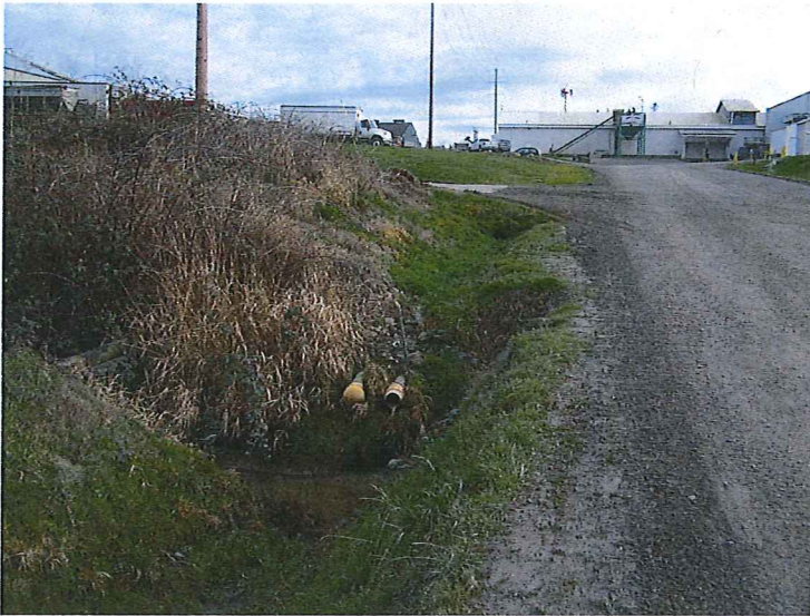
PHOTO #05 DATE: 01/16/19 TAKEN BY: JEANNE TRAN DESCRIPTION: TWO WHITE 8" PVC PIPES DRAINING THE UNLINED SHARED POND, ONE WAS CAPPED BUT THE OTHER WAS DISCHARGING. THE DISCHARGE WAS TURBID LOOKING.
