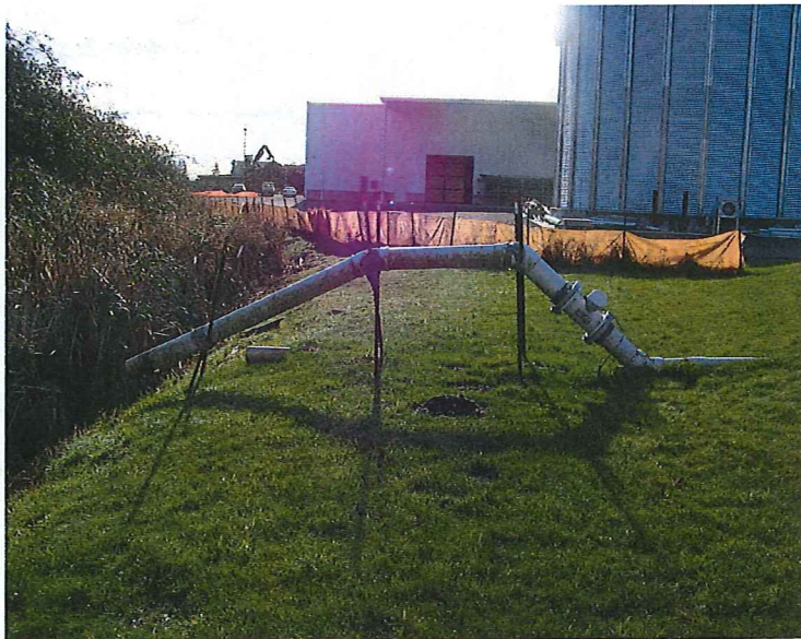
PHOTO #:17 DATE: 01/16/19 TAKEN BY: JEANNE TRAN DESCRIPTION: THIS PICTURE SHOWS THE WHITE PVC DISCHARGE PIPE WITH A FLOW METER MOUNTED ON THE ELEVATED PIPE AND DISCHARGED TO THE EXISTING DITCH WHICH FLOWS NORTHWEST UNDER ACROSS FARM TO MARKET ROAD TO LITTLE INDIAN SLOUGH.
