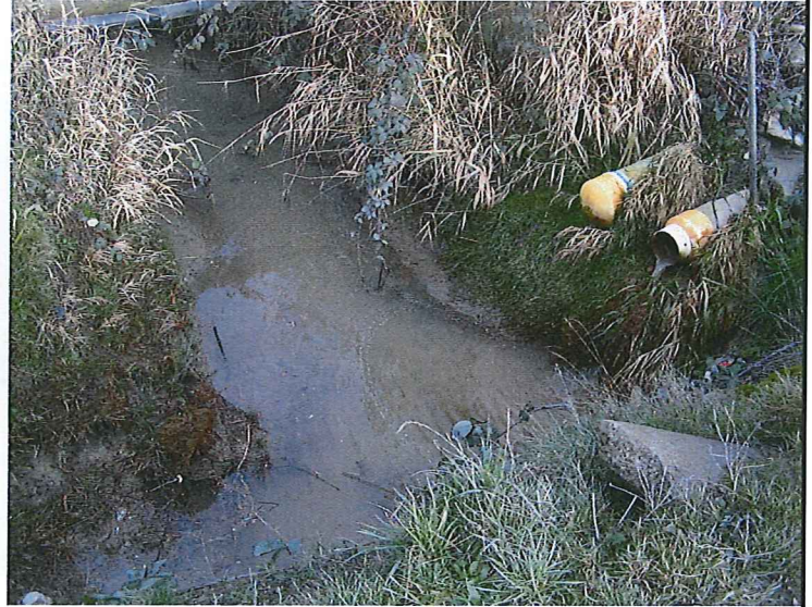
PHOTO #06 DATE: 01/16/19 TAKEN BY: JEANNE TRAN DESCRIPTION: A CLOSE UP PICTURE OF PHOTO #5, WHICH SHOWS ONE PIPE WAS CAPPED AND THE OTHER WAS DISCHARGING TURBID WATER.
