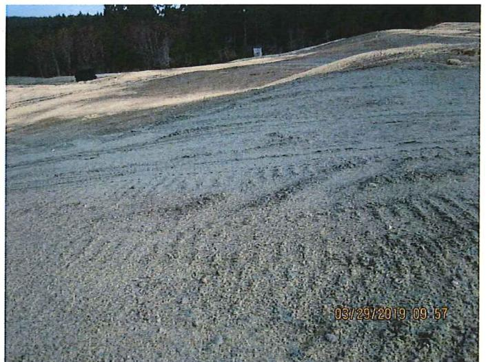
Photo 4 Description: Straw mulch is thin in areas and needs to be installed to specification: 2-3 inches thick.
