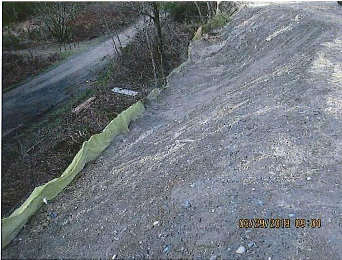
Photo 1 Description: Silt fence needs to be maintained. Slope needs to be protected with cover.
