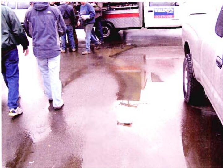
P2280399.JPG DESCRIPTION: TURBID WATER FLOWING INTO THE PARKING LOT AND DISCHARGING INTO STORM DRAIN.
