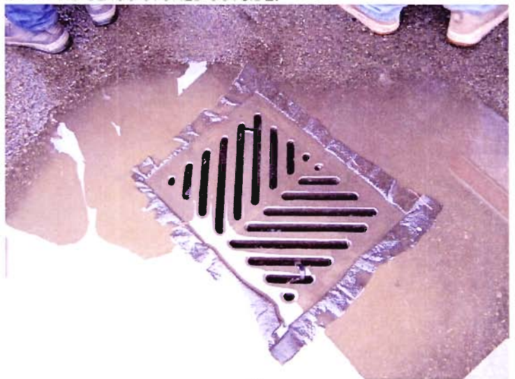
P2280400.JPG DESCRIPTION: TURBID WATER DISCHARGING TO STORM DRAIN. STORM DRAIN FITTED WITH FILTER INSERT AND OIL BOOM.
