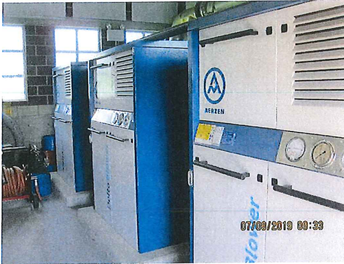
Photo 22 – Positive Displacement Aeration Blowers
