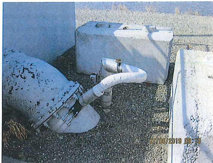
Photo 6 – Magnesium Hydroxide Injection Pipe (Smaller Pipe)
