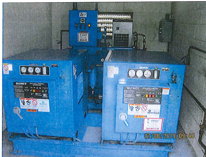
Photo 14 – Air Compressors for the Filtration System
