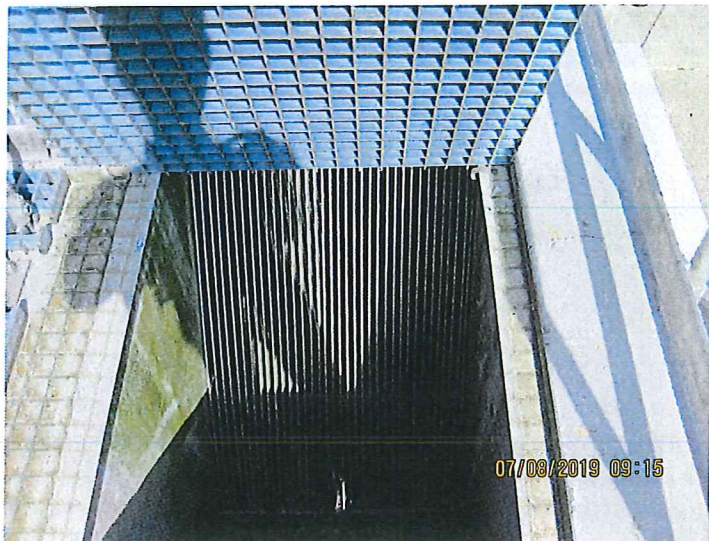
Photo 5 – Bypass Manual Bar Screen
