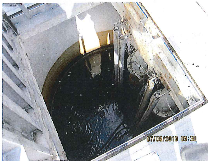
Photo 15 – Wet Well for Lagoon # 4's and Sand Filters' Effluent
