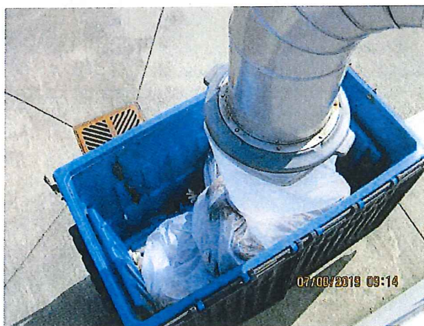
Photo 17 – Dumpster with Screenings, Rags and Grit
