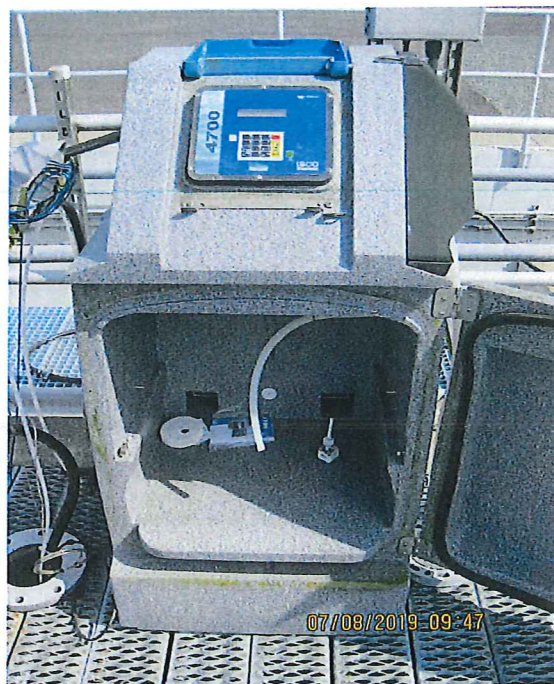
Photo 19 – Effluent Composite Sampler
