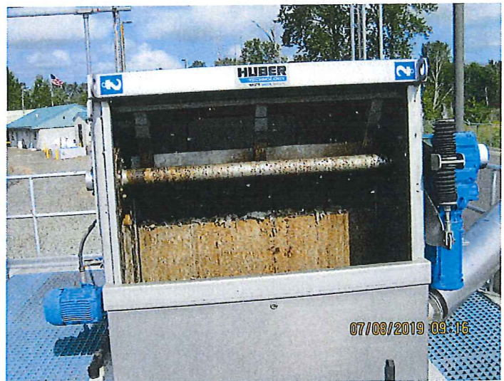
Photo 4 – Mechanical Bar Screen (Detail)
