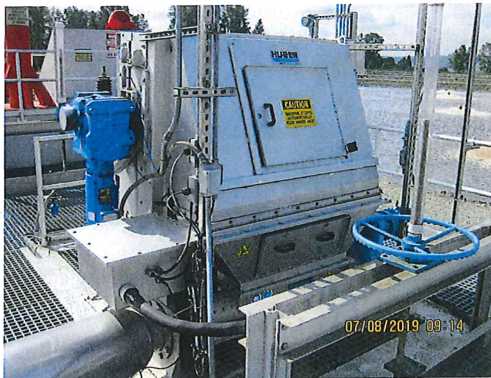
Photo 3 – 1/4-inch Mechanical Bar Screen
