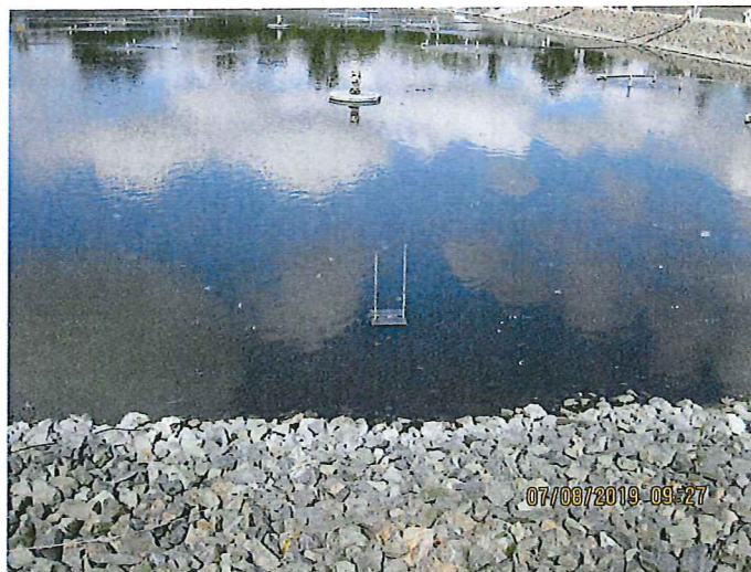
Photo 11 – Ultrasonic Unit for Algae Control (Lagoon # 3)
