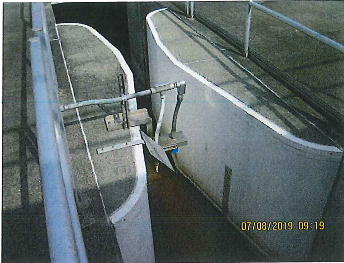
Photo 1 – Influent Parshall Flume and Ultrasonic Flowmeter
