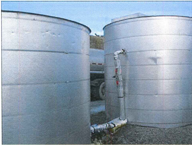
Photo 5: Tailings underdrain water treatment system tanks.
