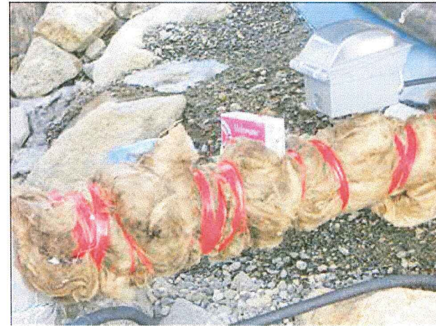
Photo 6: Insulated line running between treatment tanks at tailings underdrain water treatment system. The permittee is using a Hydroflow unit that reduces scale build-up in the treatment lines.
